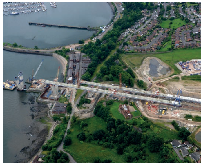
South Approach Viaduct under construction, June 2014.
