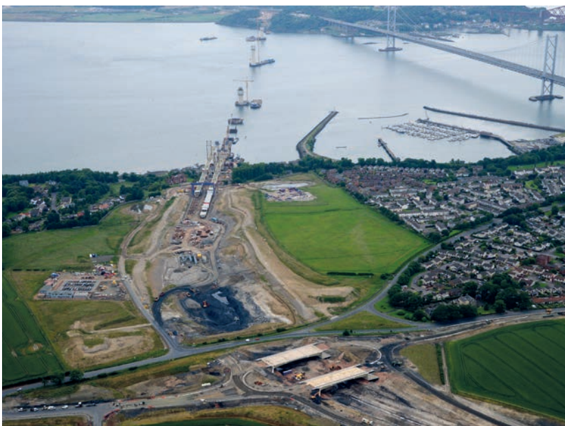
Queensferry Crossing and south approach roads under construction, June 2014.
