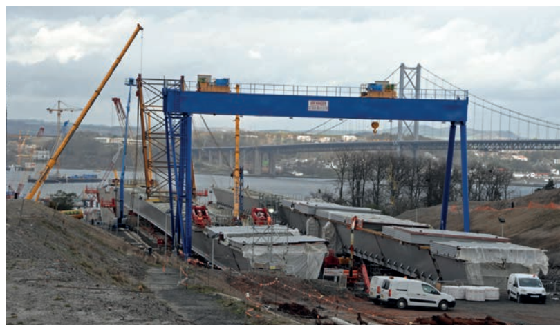
South Approach Viaduct assembly area, February 2014.
