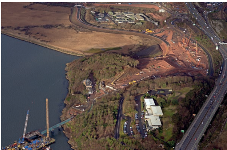
Principal Contract (north approach road) under construction, April 2014.
