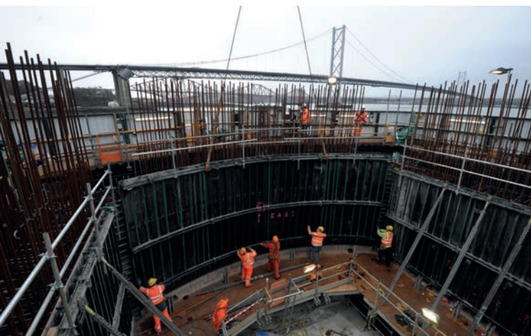
North Tower – placing reinforcement steel, February 2014.
