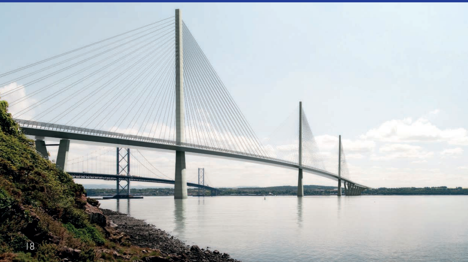
Artist's impression of the Queensferry Crossing and Forth Road Bridge.
