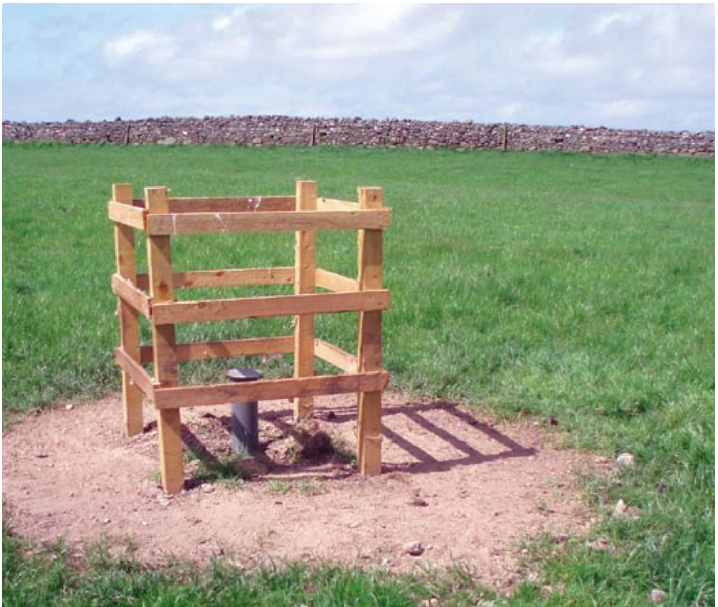
Above: Example of Piezometer insertion.
