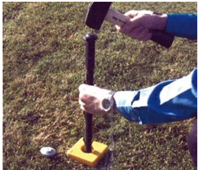
Above: Example of control point marker.
