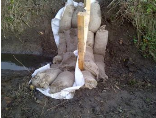
Outlet at CH600 Almond River Mainline South
