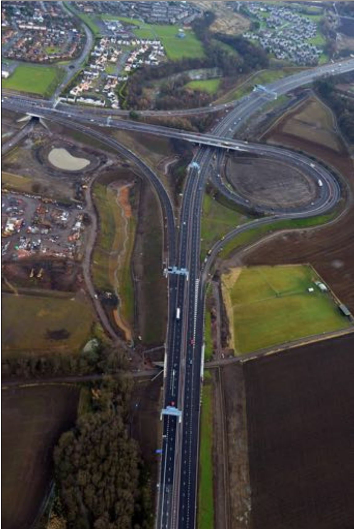
Figure 1 – Aerial view of newly completed M9J1a Junction looking eastward towards the new junction arrangement
