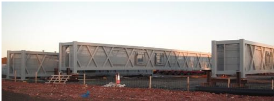
Gantry staging area
