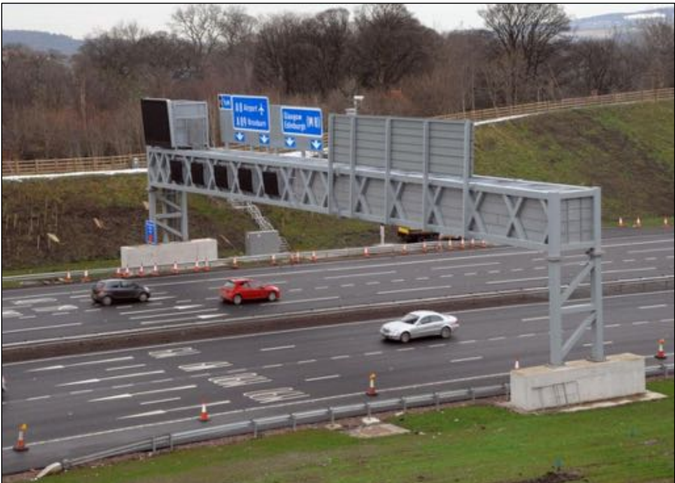
Figure 3 – Typical Completed Gantry
