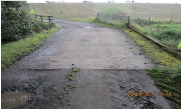
Existing watercourse crossing of Niddry Burn was utilised for works traffic
