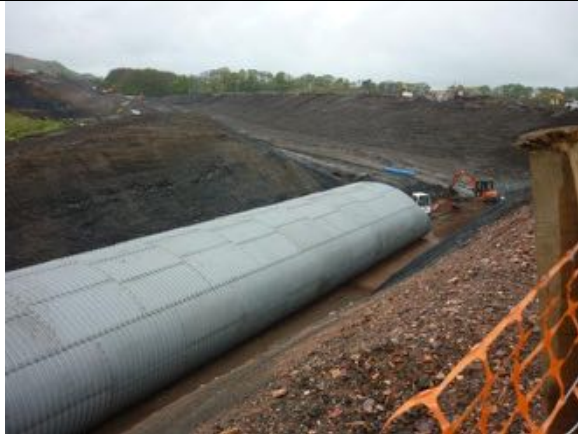
M904 New Swine Burn Culvert – corrugated structure
