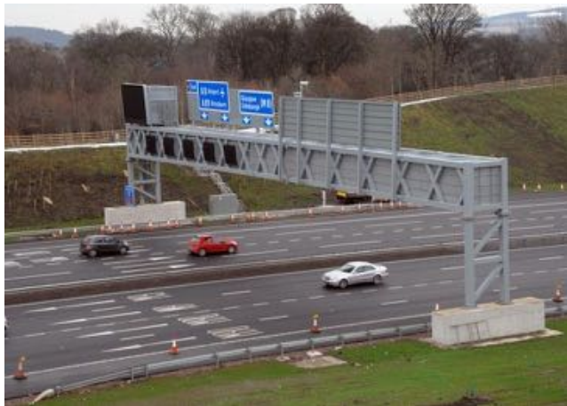
Typical completed gantry
