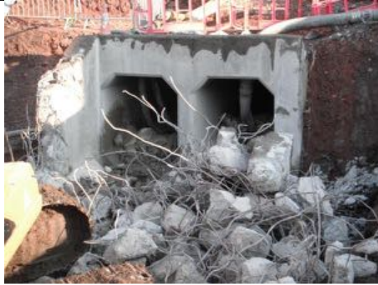
Demolition Wing walls at existing Swine Burn Culvert M907E
