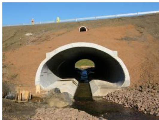
M904 New Swine Burn Culvert
