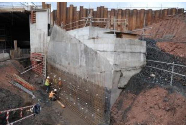
Structure M905E Overton Road – Demolition of Wing walls
