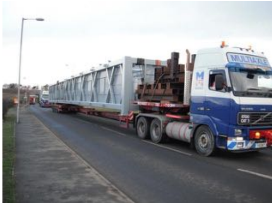
Prefabricated gantry delivery to site 16 th February 2012
