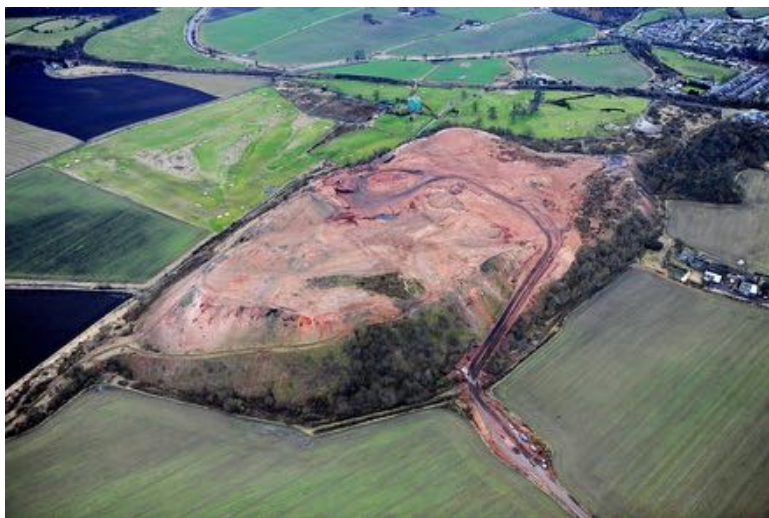
Niddy Bing (operated by Hunter Demolition) – a source of reusable waste from previous oil shale extraction industry
