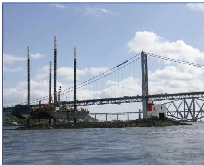
• Marine investigations in Firth of Forth
