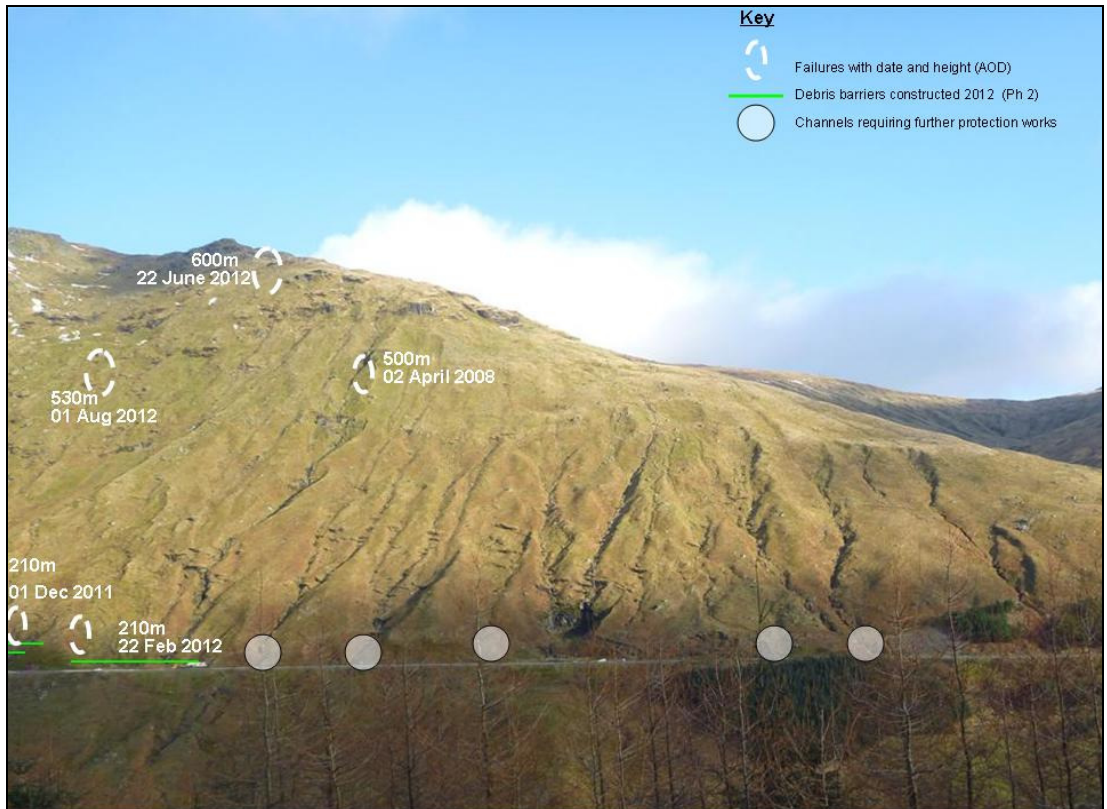
Figure 2-4: Image showing recent slope failure locations and location of existing and proposed debris barriers. Image courtesy of Scotland TransServ
