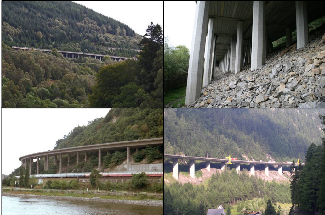
Figure 6-4: Example of viaducts on side-long ground – A9 Killiecrankie (top left and top right); Rhine Valley Krahenberg Bridge (bottom left), and; Brenner Autobahn Lueg Bridge (bottom right)
