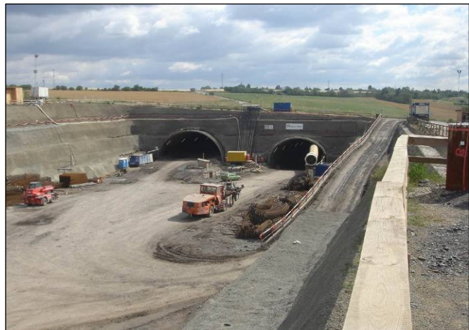
Figure 6-5: Twin bore road tunnel portal during construction – Photo courtesy Hochtief AG
