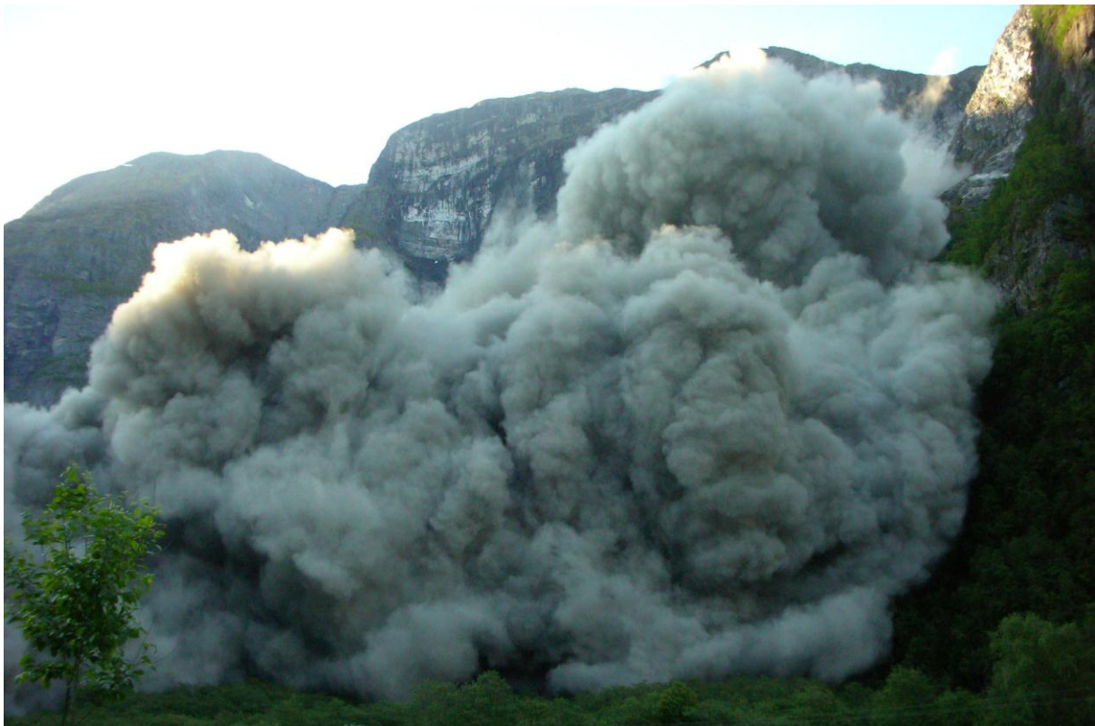
Figure 5. Dust cloud caused by blasting at Skjerpung, Norway in 2010. The cloud travelled around 7km down the valley and fjord of Nærøydalen. (Photograph by Paulsen, courtesy of Ulrik Domaas, Norwegian Geotechnical Institute.)
