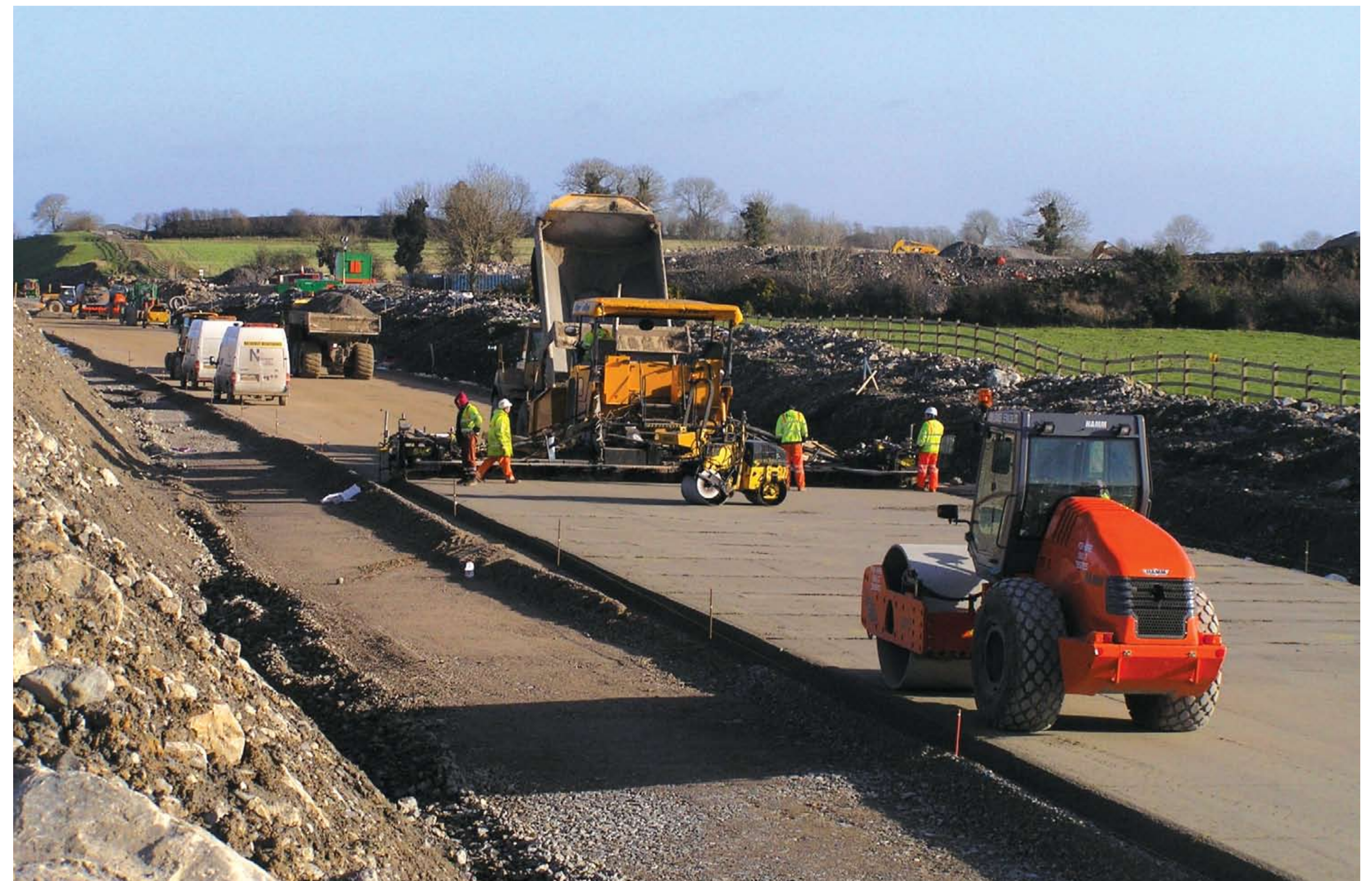
ROAD CONSTRUCTION WORKS
