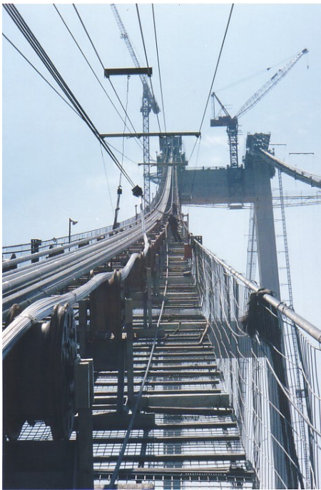
Figure C9 - Jiangyin Suspension Bridge Main Cable (PPWS Method)
