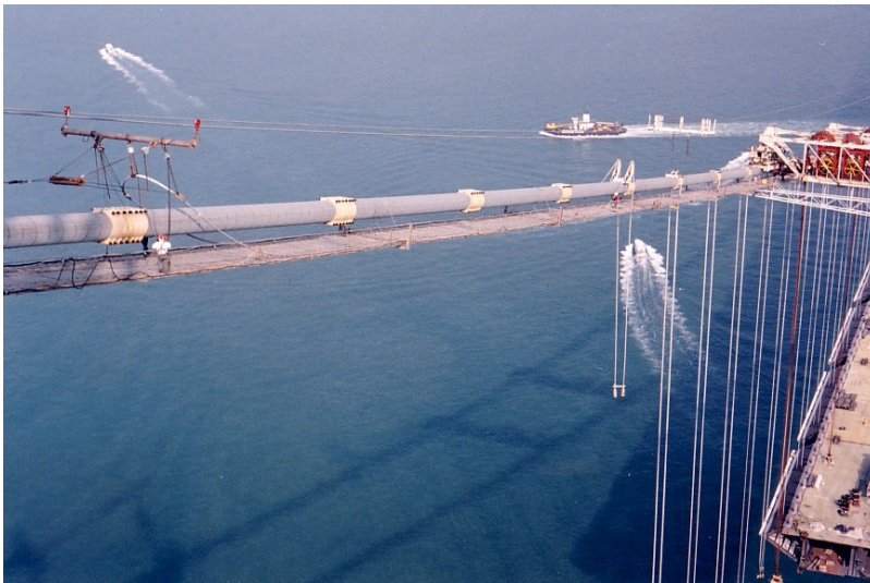
Figure C8 - Tsing Ma Suspension Bridge Main Cable (Aerial Spun Method)
