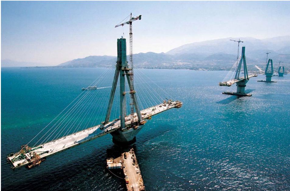
Figure C17 – Rion Bridge – Deck and Cable Stays Under Construction
