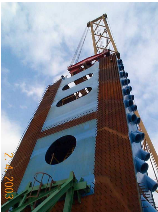
Figure C16 – Rion Bridge Prefabricated Tower Section
