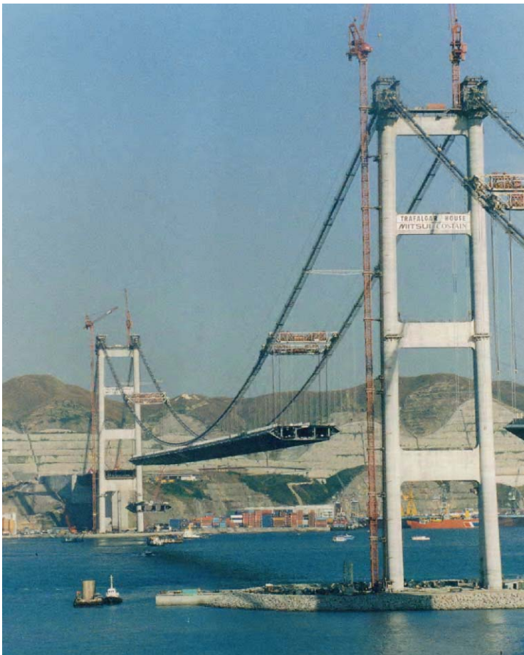
Figure C11 – Lifting Deck Panels at Tsing Ma Suspension Bridge
