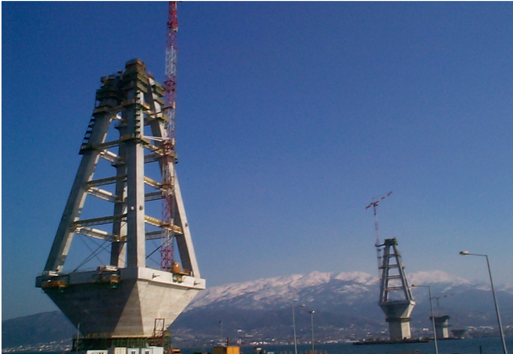
Figure C15 – Rion Bridge Towers under Construction
