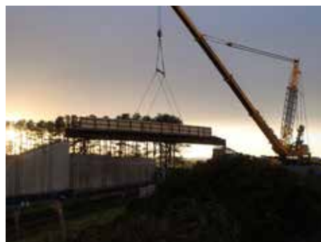
Top left Ground works, M8
