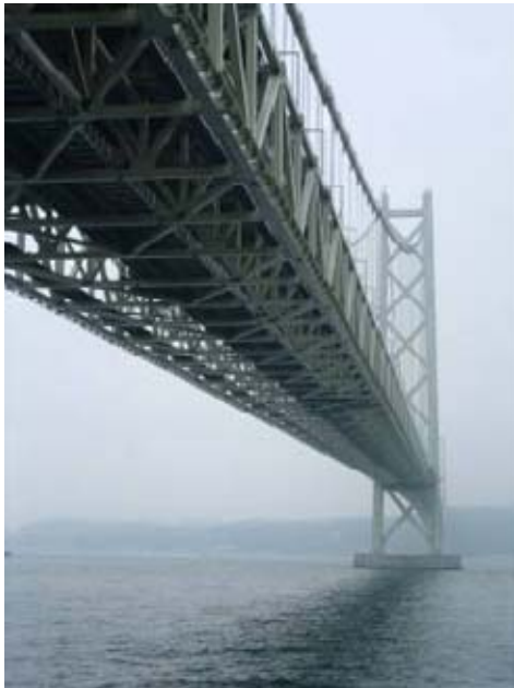
Figure: A.1 Akashi Kaikyo Bridge
