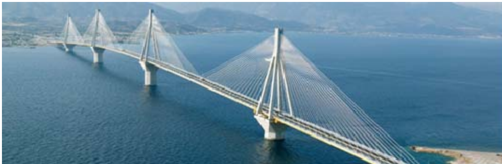
Figure: A.7 Rion-AntiRion Bridge, Greece
