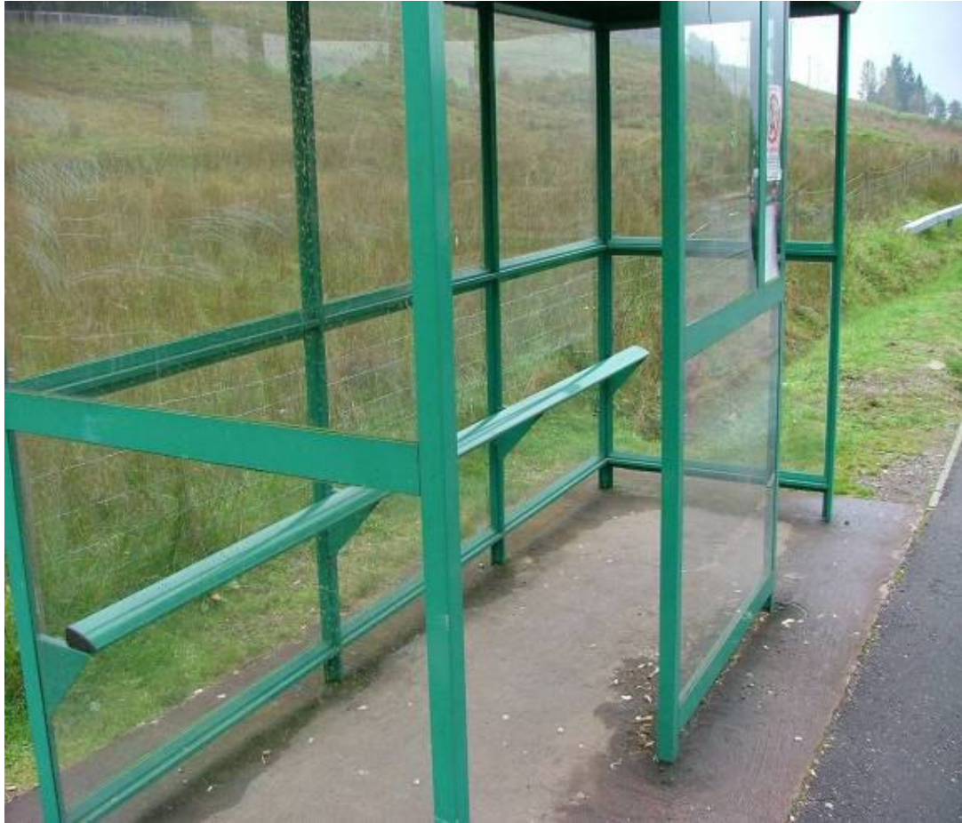
Bus shelter with narrow 'perched rail' seating
