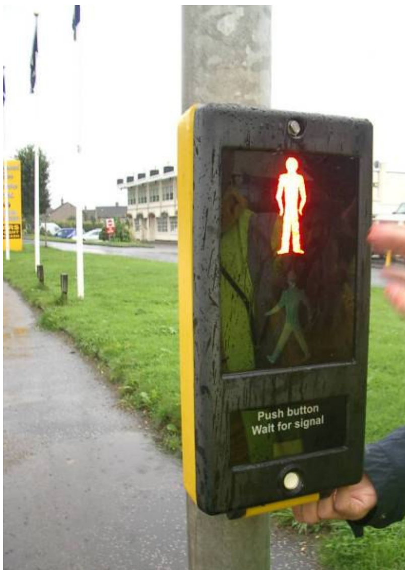
Controller with red/green man symbols and tactile rotating cone but without large push-button
