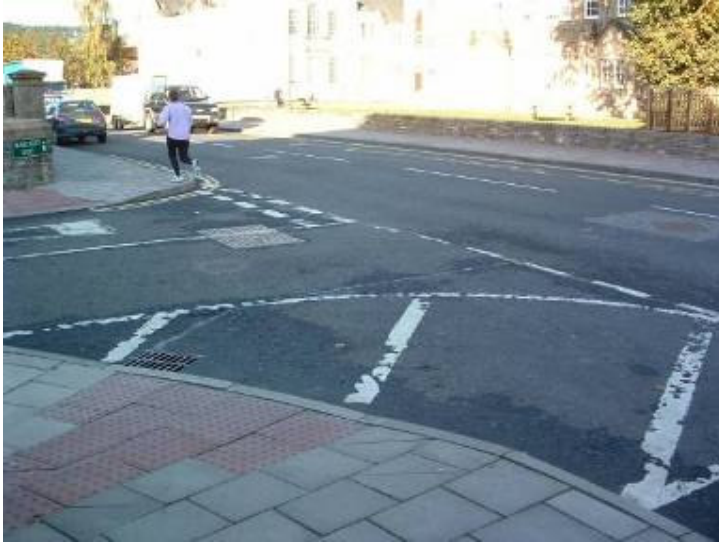
Incorrectly installed tactile paving
