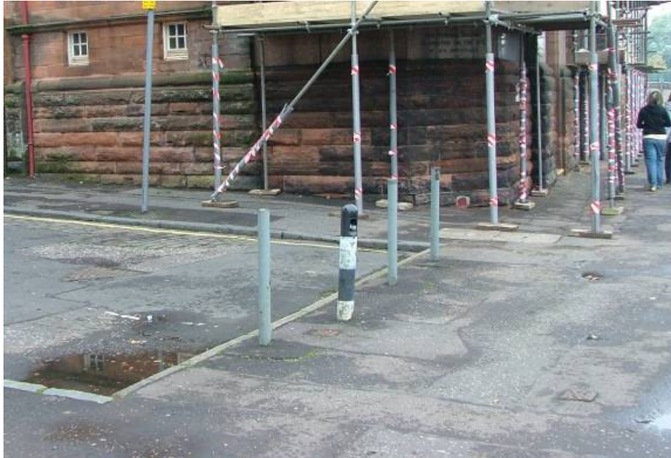
Bollards lacking colour contrast and scaffolding obstructing the pavement
