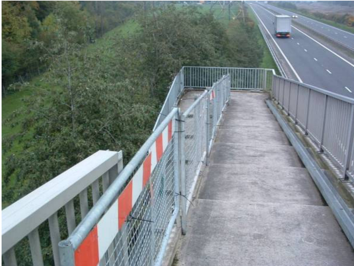
Stepped ramp unsuitable for wheelchairs
