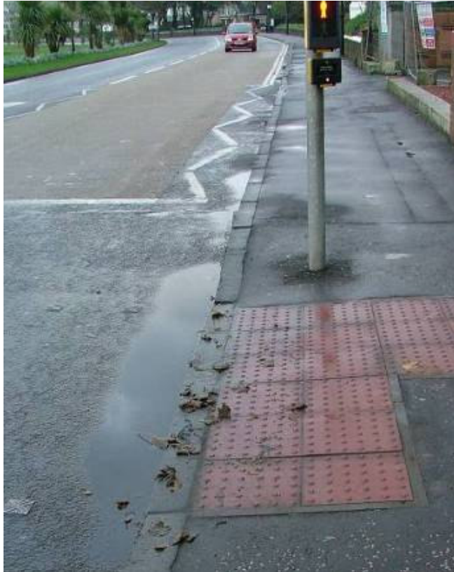
Poor drainage causing ponding at a crossing point
