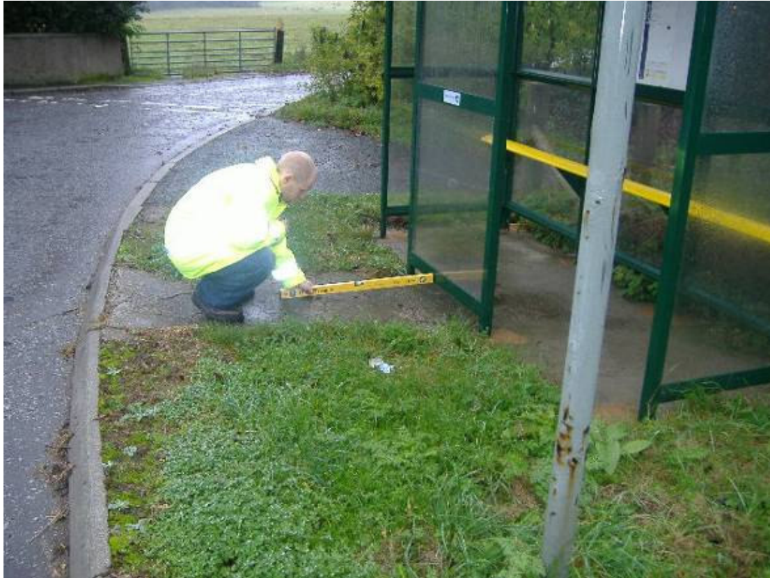
Inaccessible bus shelter with no raised boarding kerb
