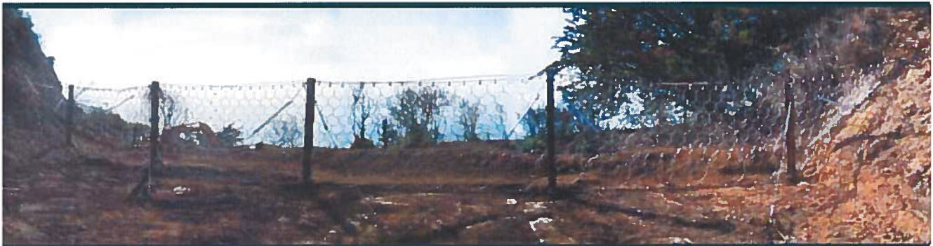
Completed Debris Flow Barrier
