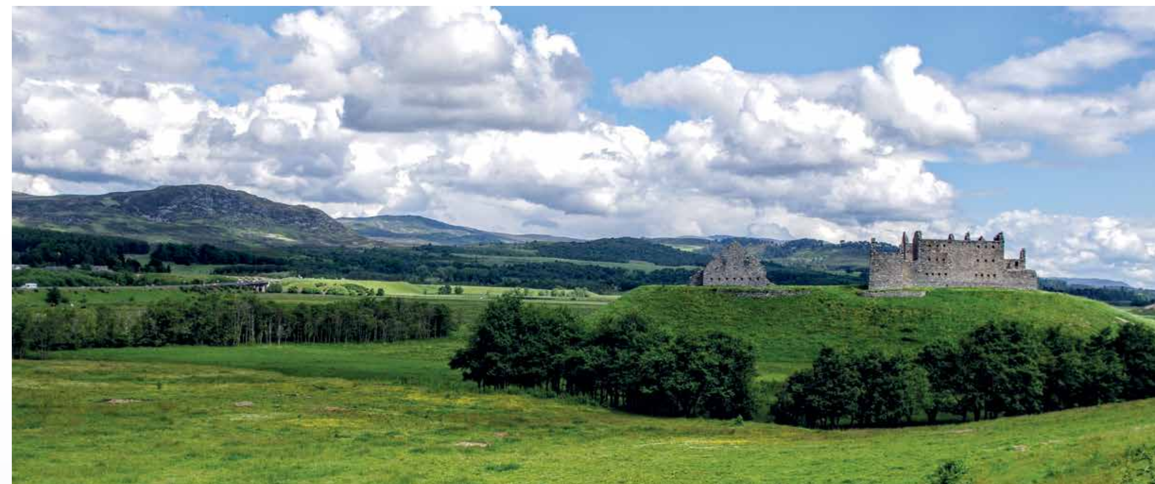
Ruthven Barracks near the A9
