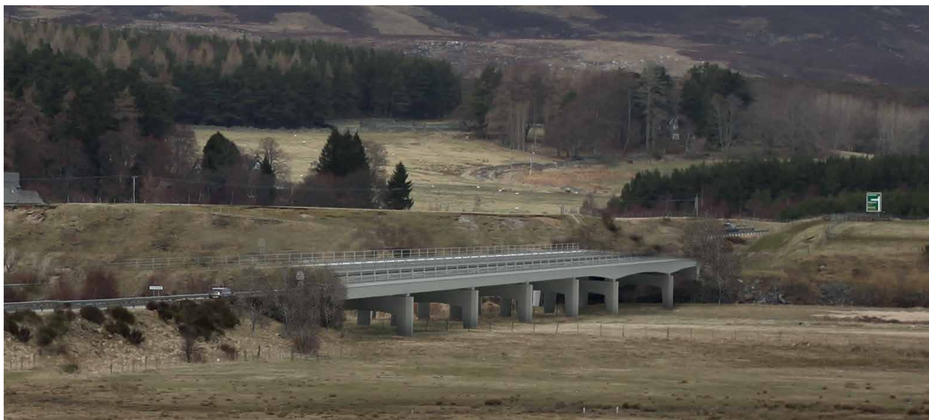
Example of bridge similar to existing
