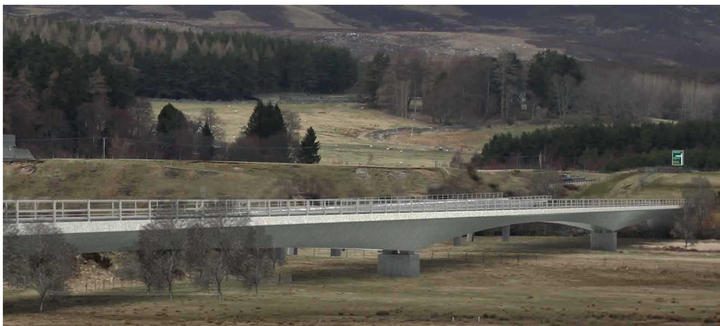
Example of steel/concrete bridge supported by piers
