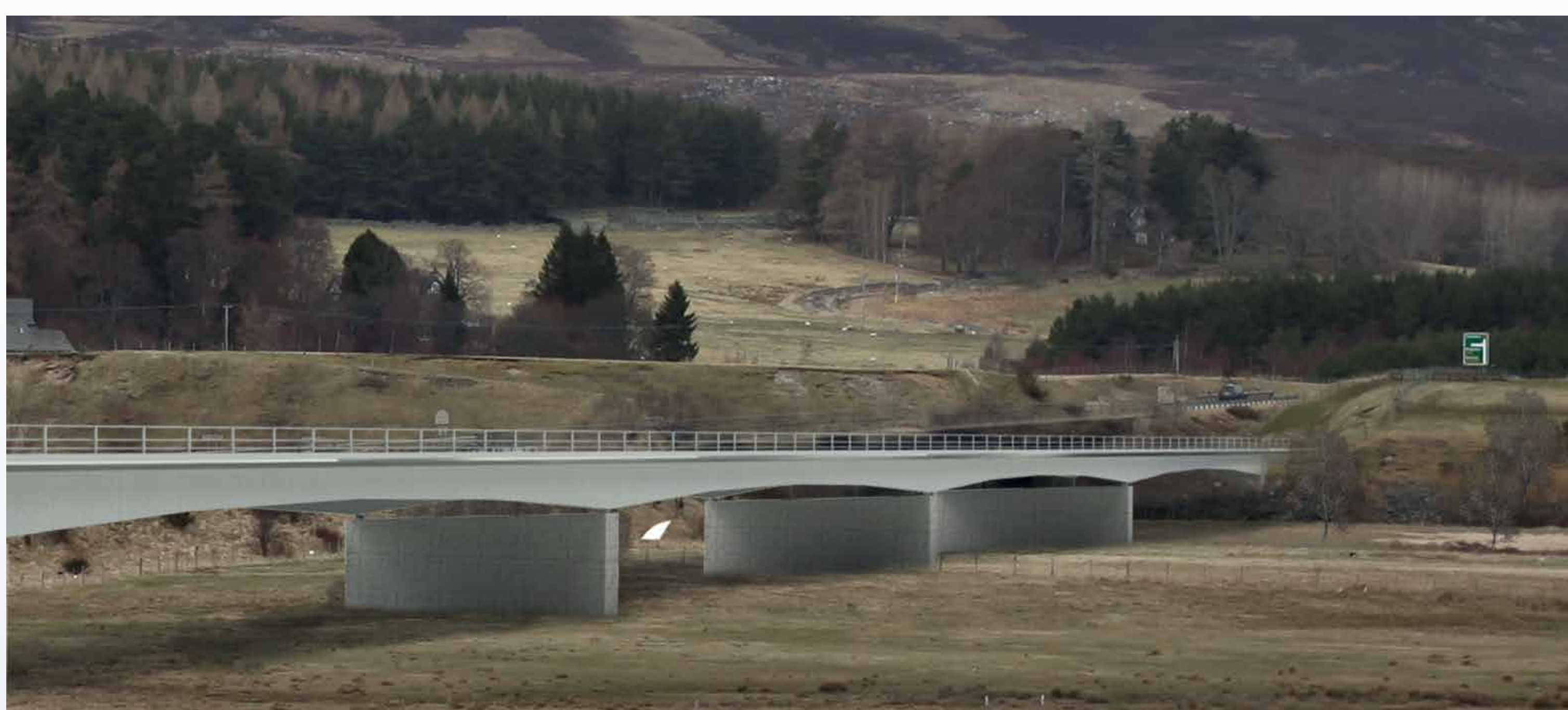
Example of steel/concrete multi-span viaduct
