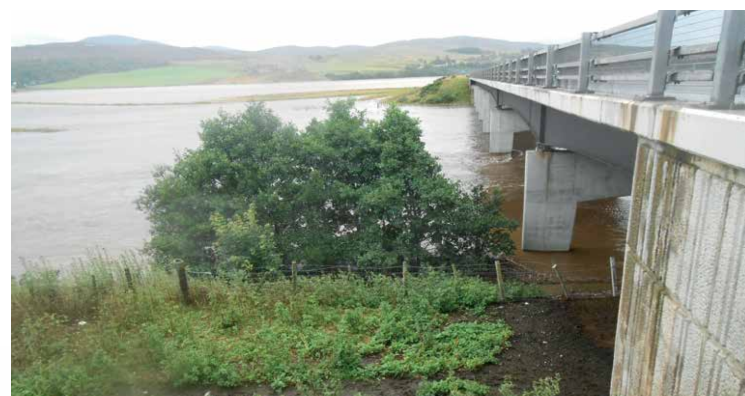
View of flooding at River Spey, looking south across Insh Marshes towards Ruthven Barracks, August 2014
