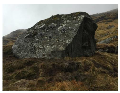
Figure 2.1 - Large boulder stabilised in situ on Beinn Luibhean
