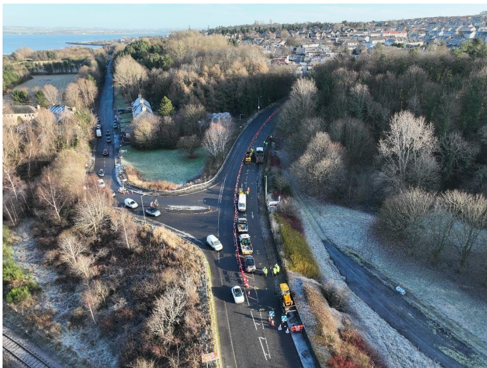
Figure 17: the A904/A993 road corridor undergoing works, where the layout changes support future improvements for active travel along a route bordered by woodland.
