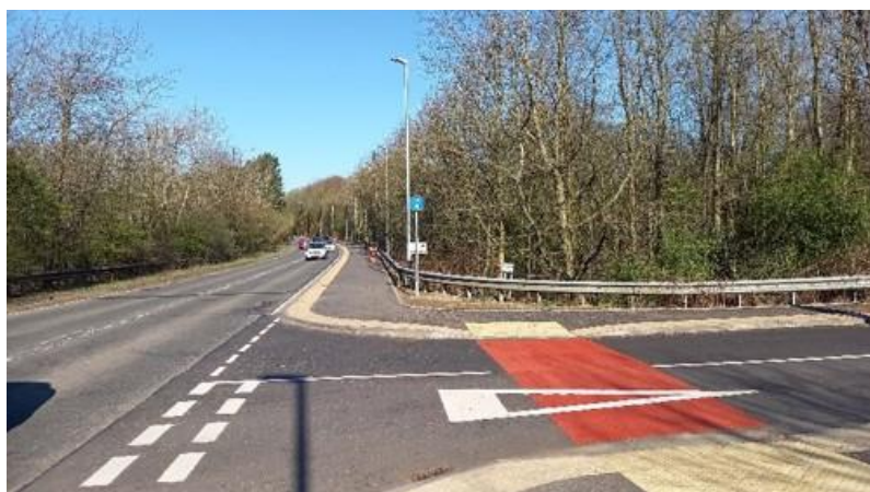
Figure 9: a junction after interventions. A drop kerb on either side of the road has been constructed and a red surfaced crossing.
