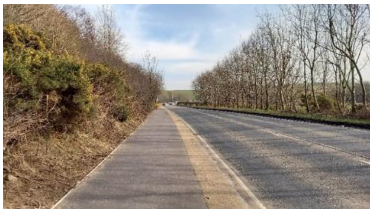
Figure 7: the A807 improvements after intervention showing a newly constructed pavement.
