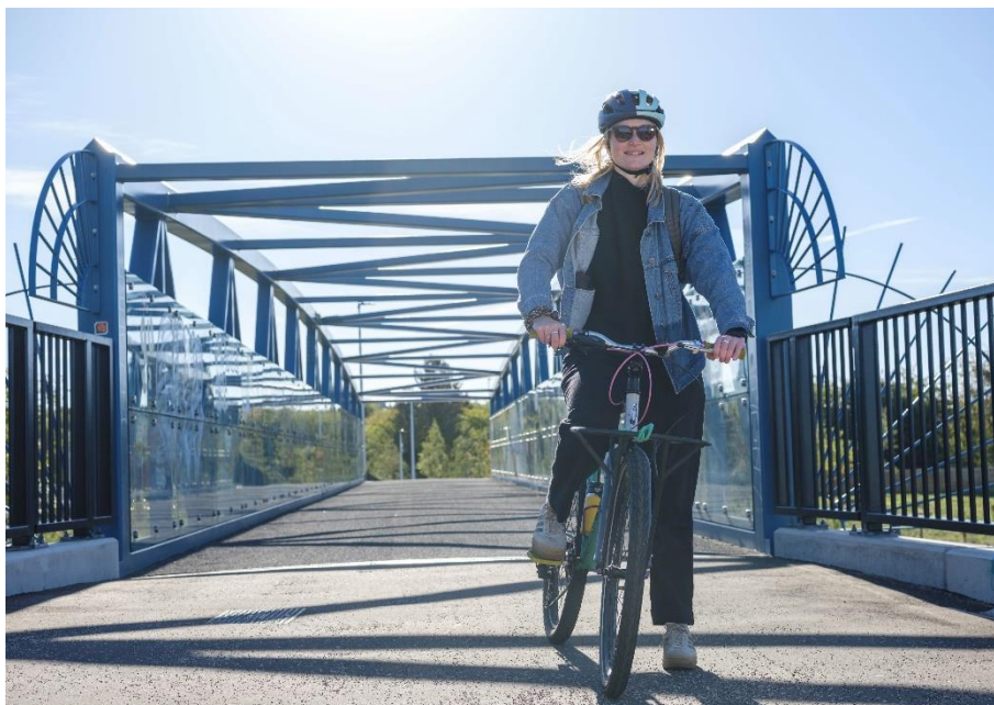
Figure 11: a cyclist crossing the new bridge between Roseburn and the Union Canal.
