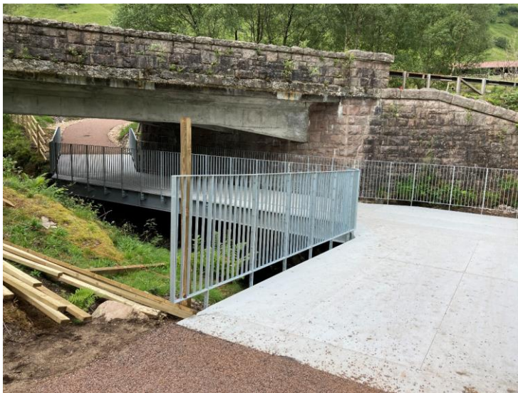
Figure 13: a new pedestrian bridge across a river beneath the A82.
