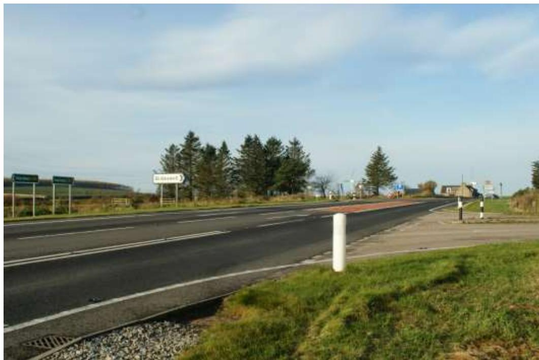
**Figure 4.2.9 Ghost Island staggered junction at Saddle Hill**
