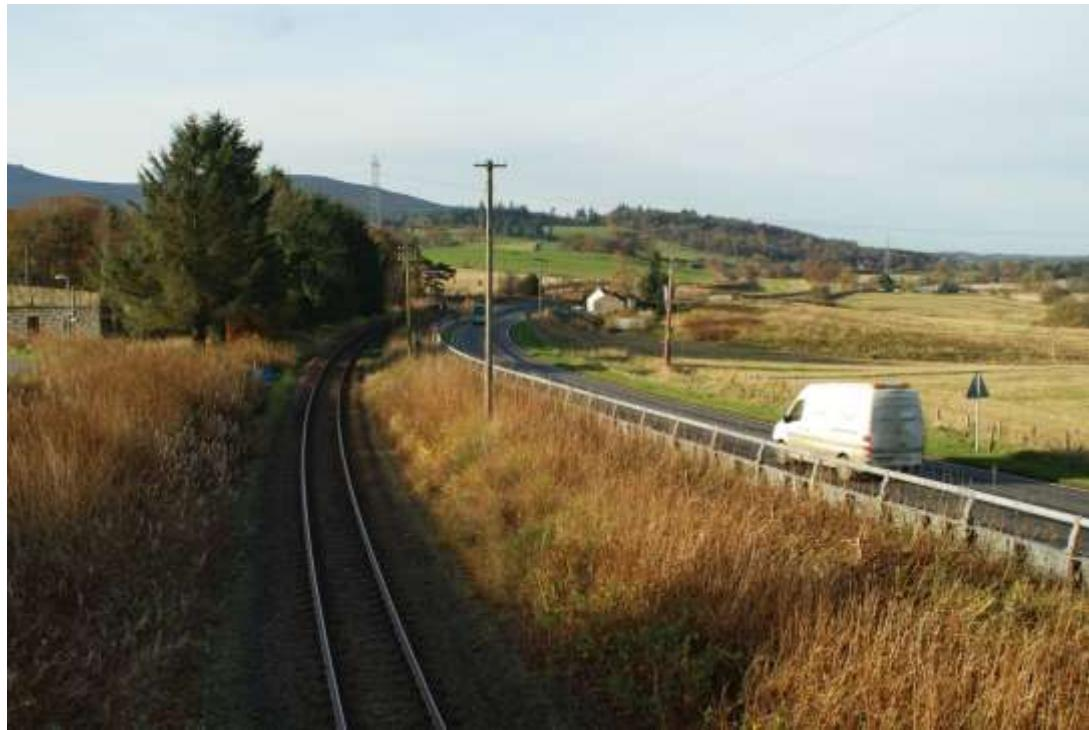
**Figure 4.2.21 High Containment Barrier adjacent to Aberdeen to Inverness Railway Line near Pitcaple.**
