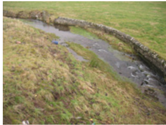
Plate 2: Bank protection upstream of the Annfield Bridge.
