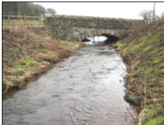
Plate 3: The old bridge carrying the D4715 over the Headshaw Burn.
