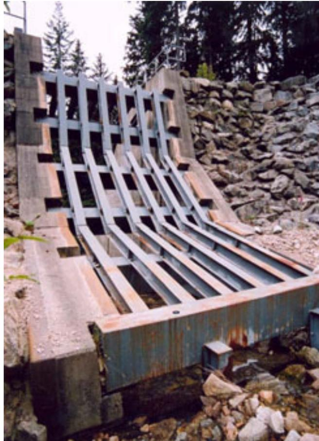
**Figure 8.11 – Downstream drainage outlet of debris basin, Mackay Creek, North Vancouver, British Columbia, Canada. The black disc visible on the base of the structure is 72mm in diameter.**
