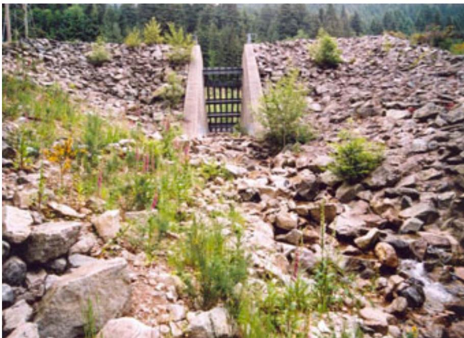
**Figure 8.10 – Debris basin showing the downstream barrier and drainage outlet, Mackay Creek, North Vancouver, British Columbia, Canada.**
