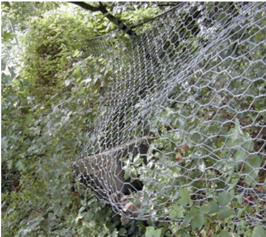
**Figure 8.20 – Flexible fence with a fallen rock that has been successfully arrested, Abbey Craig, Stirling.**
