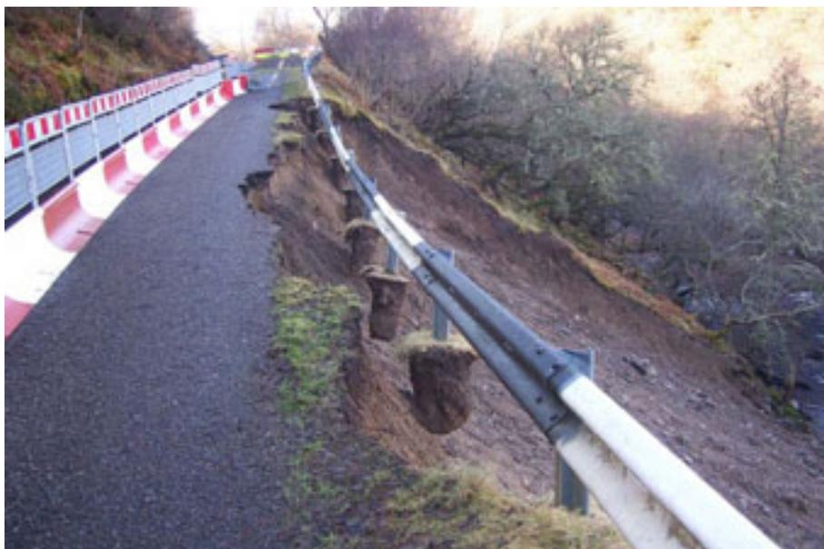
**Figure 2.24 – Torboll, showing ongoing erosion, 14 February 2007.**
