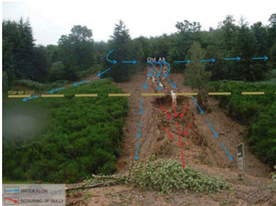
**Figure 2.6 – Influence of old road on debris flow at A9 Dunkeld. The central flow is shown and the northern flow can also be seen on the left of the picture. Photograph dated 11 August 2004. (Courtesy of Alan Mackenzie, BEAR.)**
