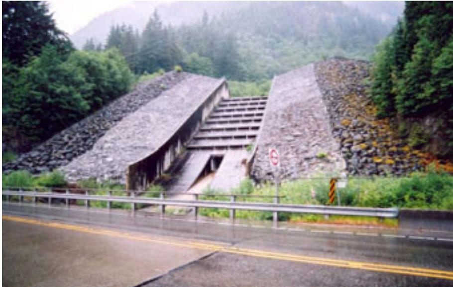
**Figure 8.12 – Concrete spillway on the downstream face of a debris basin barrier, Charles Creek, Sea-to-Sky Highway, British Columbia, Canada. The drainage outlet may be seen in the centre of the spillway.**
