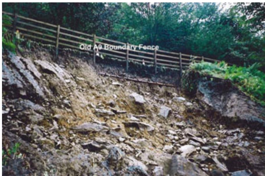
**Figure 2.7 – Instability at the downslope edge of the old A9 above the central debris flow. Photograph dated 12 August 2004. (Note that the brown pipe running horizontally across the backscarp is a telecommunications duct.)**
