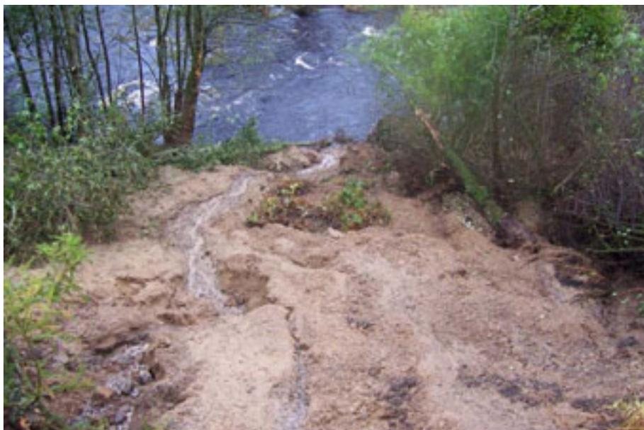
**Figure 2.27 – Erosion and deposition below road, Struie.**
