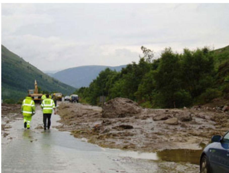
**Figure 2.3 – Debris fan containing boulders (estimated up to 9 tonnes) at A83 Cairndow.**
