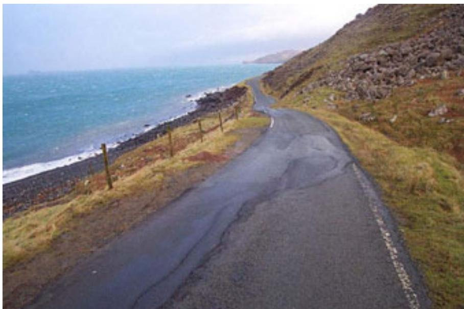
**Figure 2.17 – Road at Duntulm, Skye being moved by mass movement of boulder field, accelerated by erosion at toe**
