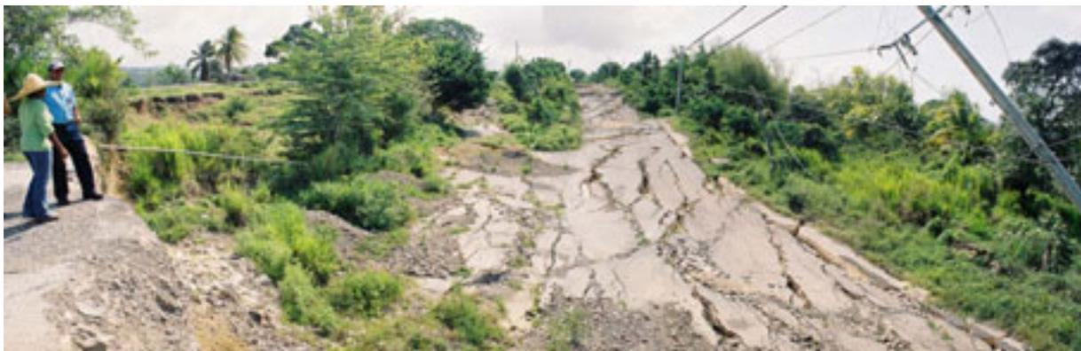
**Figure G.16 – Deep rainfall induced landslide on the A2 road between Whitehall and Martins in St Mary Parish, eastern Jamaica.**
