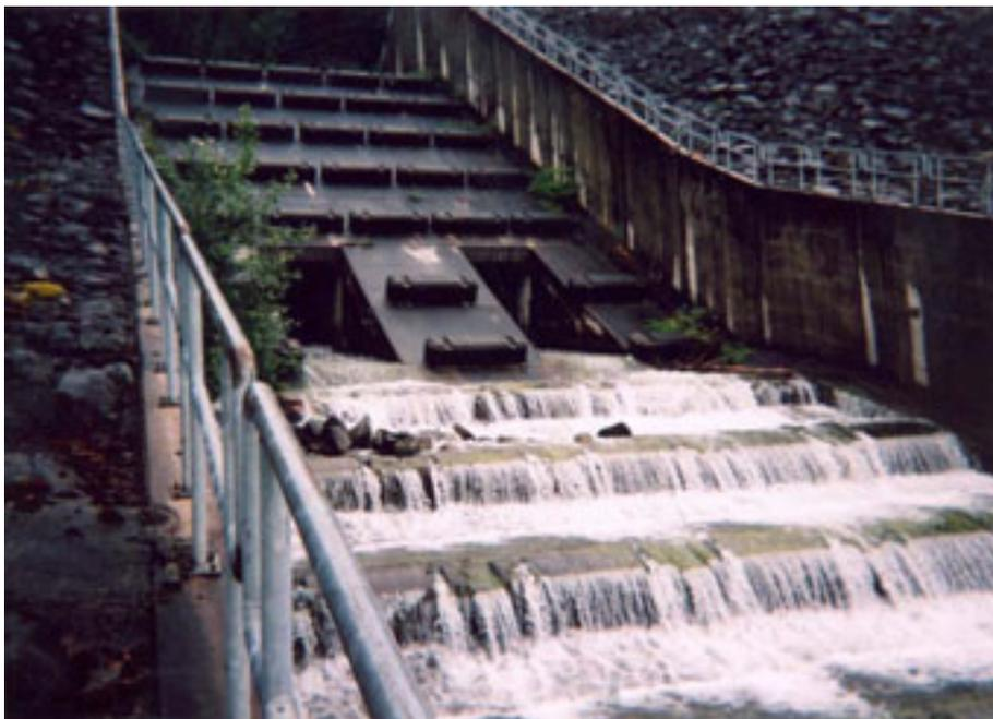
**Figure 8.13 – Detail of a concrete spillway on the downstream face of a debris basin barrier, Harvey Creek, Sea-to-Sky Highway, British Columbia, Canada. The drainage outlet may be seen in the centre of the spillway.**
