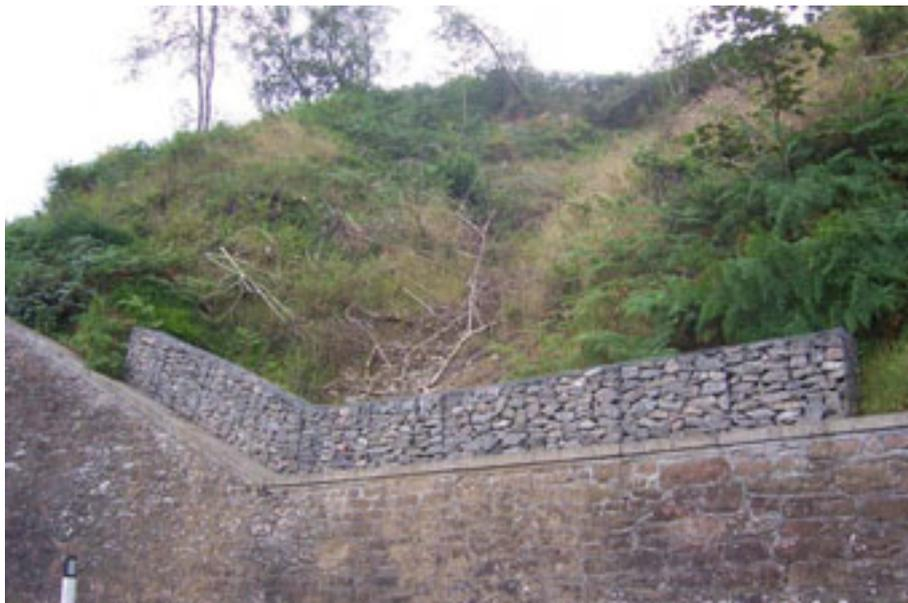
**Figure 2.28 – Gabion debris trap, Struie.**
