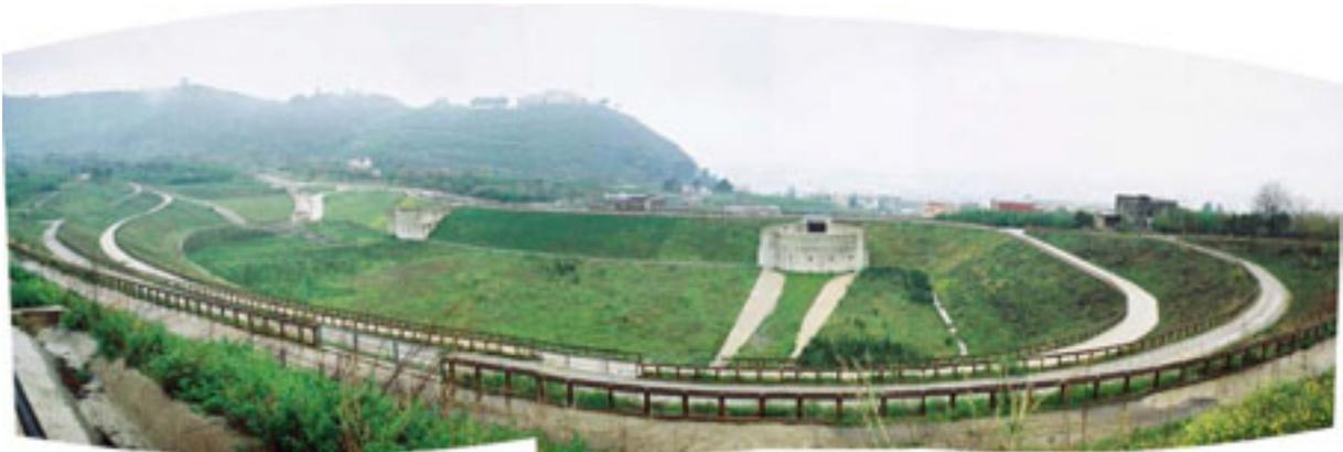
**Figure 8.21 – Debris basin with a capacity of approximately 176,000m<sup>3</sup> at Sarno in Italy.**
