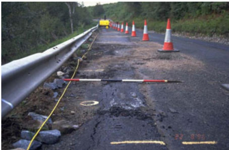
**Figure 8.23 – Deformation of the A86 carriageway alongside Loch Laggan due to a series of minor landslides.**
