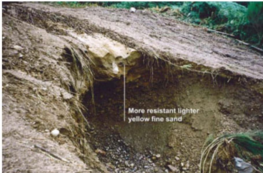
**Figure 2.8 – The top of the central erosion gully at the top of the cut slope. The overhang of the denser yellow fine sand is clearly visible and it appeared that this material was better able to shed the water and debris. Photograph dated 12 August 2004.**
