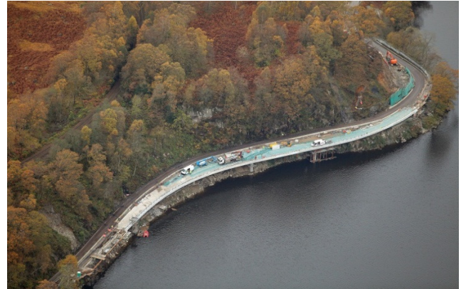
Figure 1.4: Pulpit Rock improvements under construction
