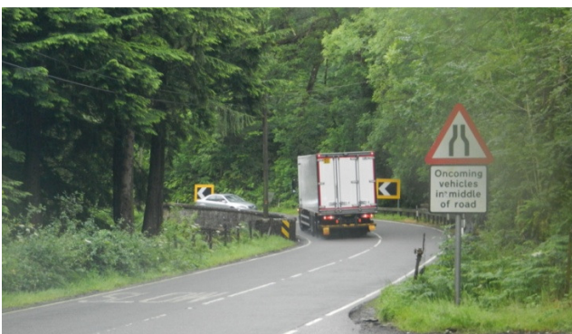
Figure 2.3.8: Poor visibility on Inveruglas Water Bridge
