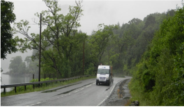
Figure 2.3.23: Overhead telecoms in eastern verge
