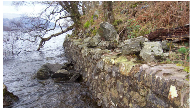
Figure 2.3.18: A82 400 W56 Coire Nan Each Retaining Wall
