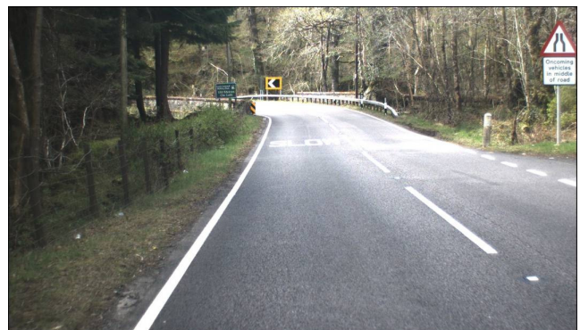
Figure 2.3.2: A82 southbound approaching Inveruglas Water bridge
