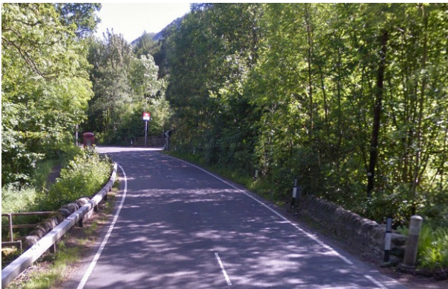
Figure 2.3.19: Double pipe culvert by the A82 423F Ardlui Footbridge
