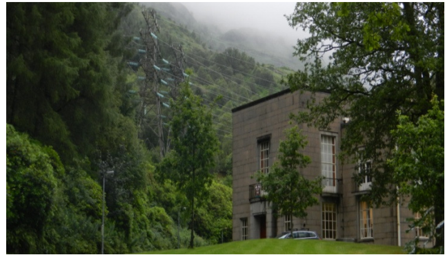
Figure 2.3.22: Transmission Lines at Sloy Power Station
