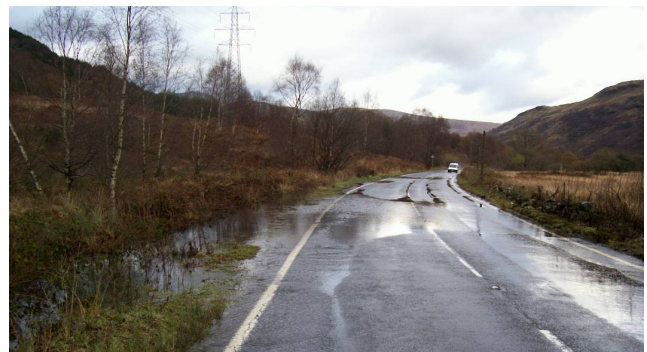
Figure 2.3.20: Flooding on the A82 at Garabal
