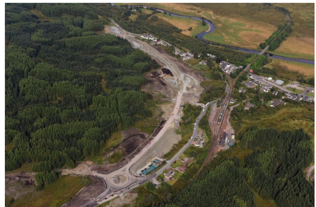
Figure 1.5: Crianlarich Bypass under construction
