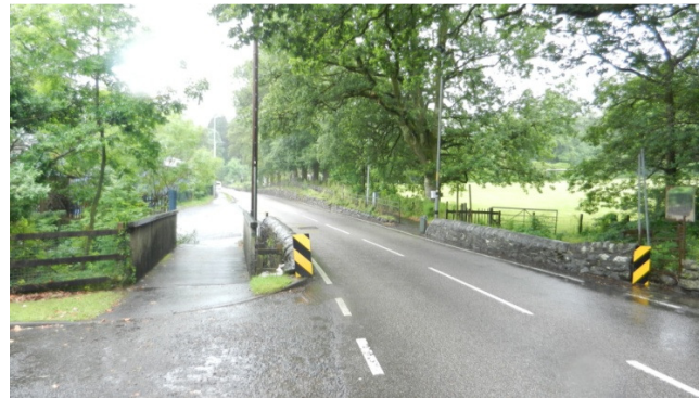
Figure 2.3.6: Tarbet bridge and pedestrian bridge
