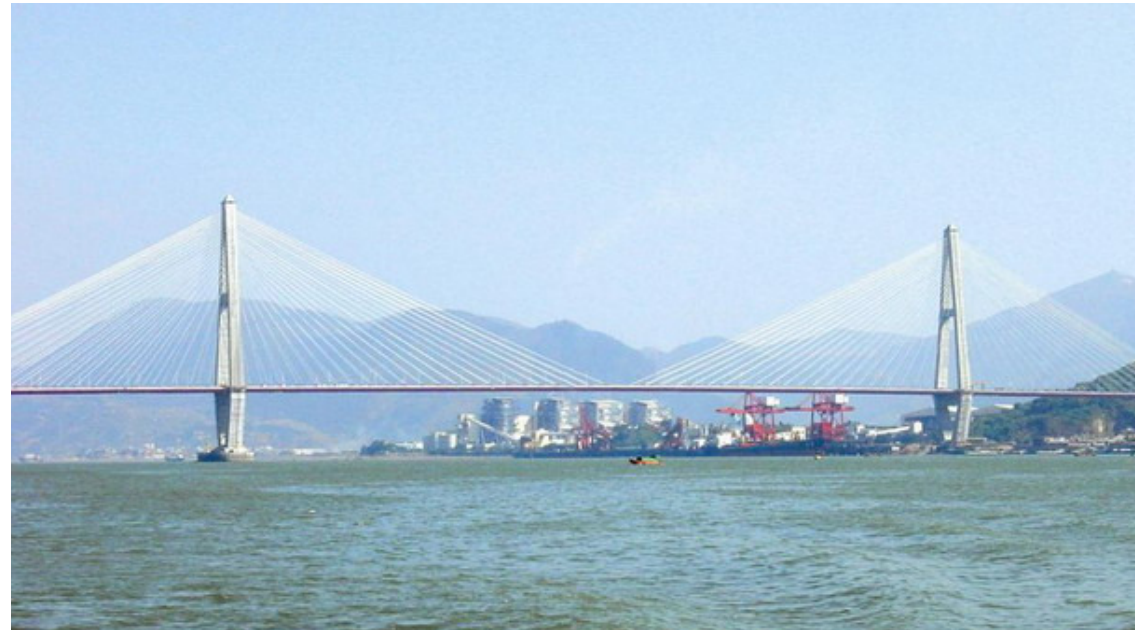
Ching Chau Min Jiang Bridge, Fuzhou, China
