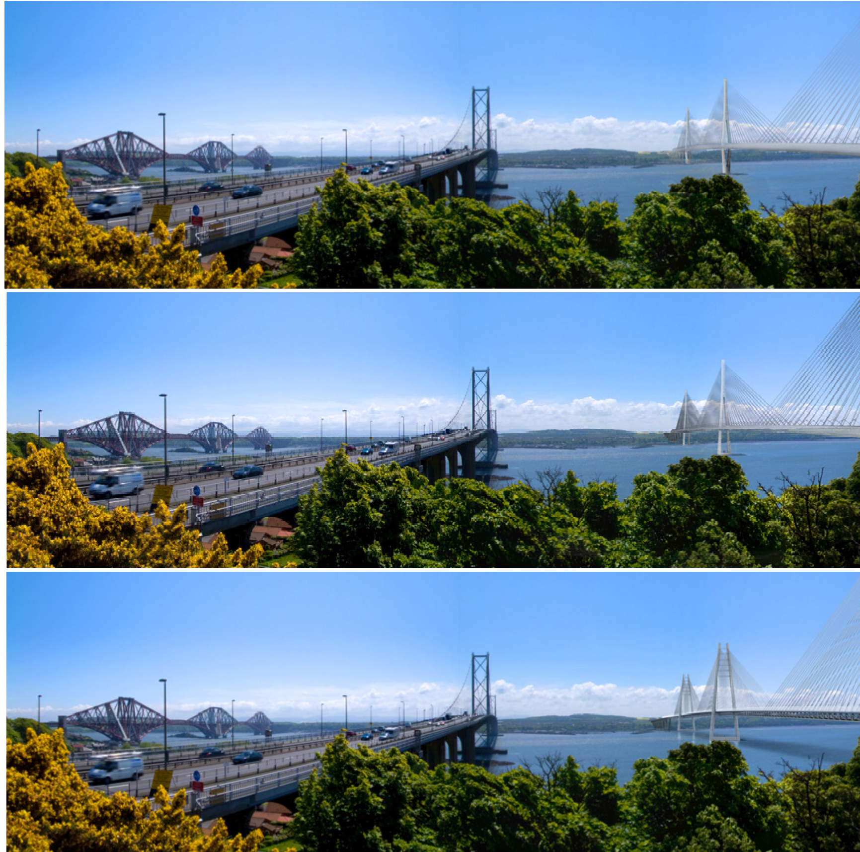
Figure C.19 Comparison Needle Tower, Inverted Y Tower and H-shape Tower
