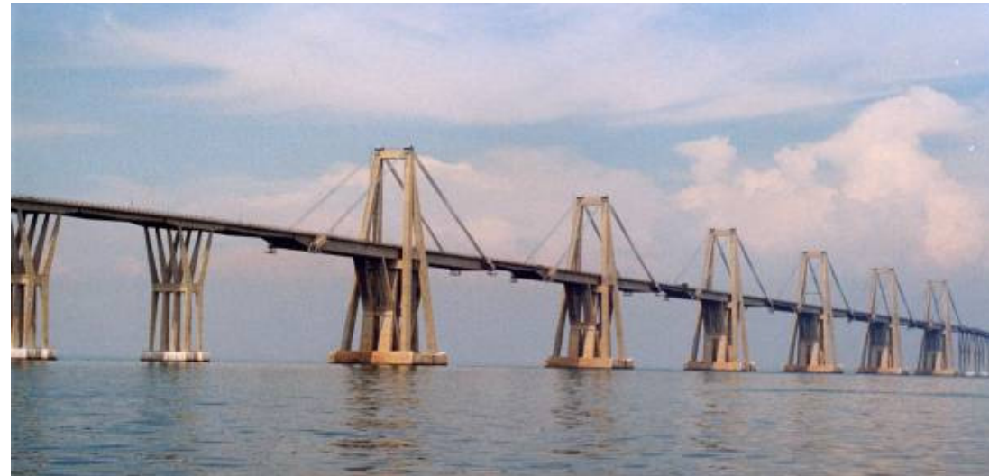
Maracaibo Bridge (1962), Venezuela
