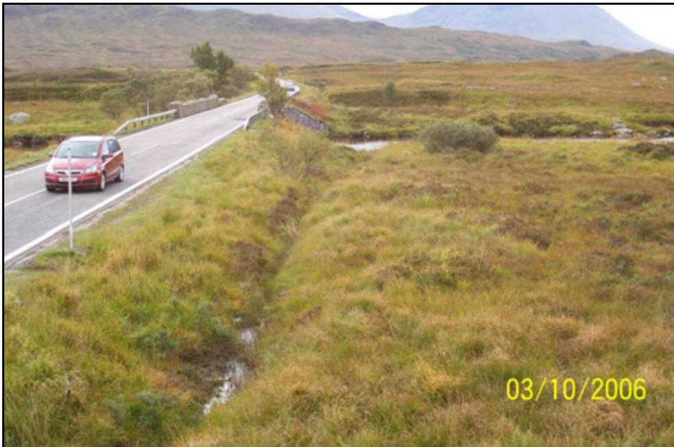
**Figure 6.1 Road raised on embankment**
