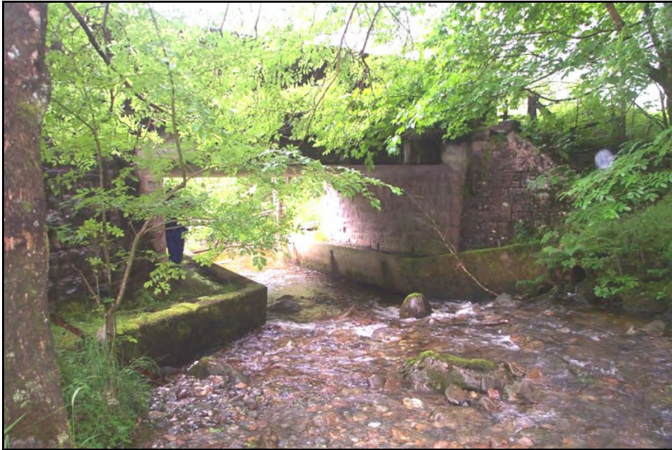
Figure 3.1 View looking downstream to Allt Fhiodhan Bridge, note the reduction in channel capacity and the presence of the riffle within the concrete foundations immediately upstream of the bridge.
