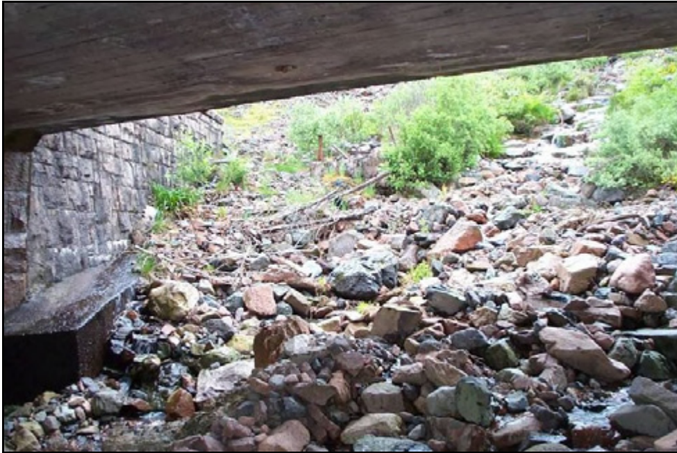
Figure 3.3 View looking upstream from under the Alltanrigh Bridge.
