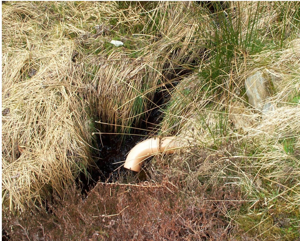
Photograph A1: Septic tank discharge pipe into local burn (feature 2.4) – looking west from location NN 38356 25323
