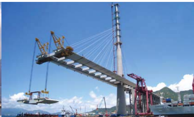
Installation of deck sections on a cable-stayed bridge.
