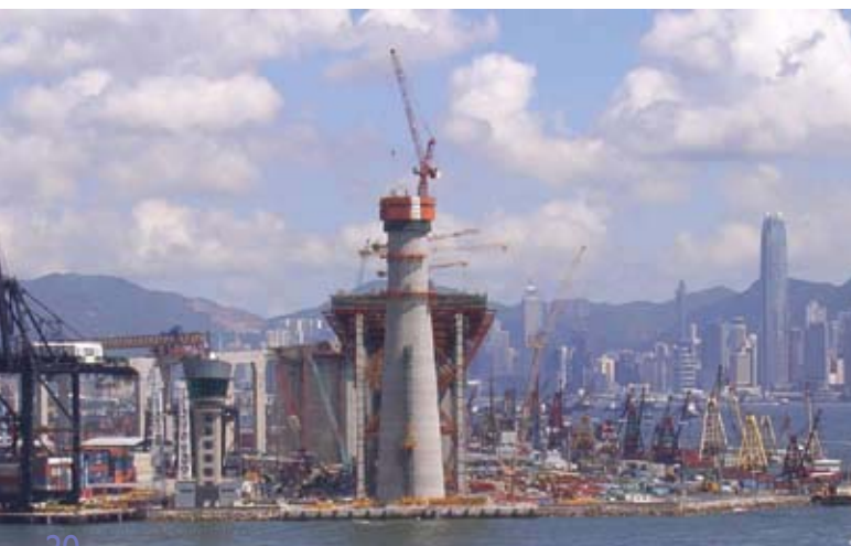
Construction of a mono-tower for a cable-stayed bridge
