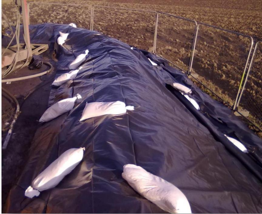
**Figure 3: Stockpiles covered to prevent deterioration of soils**
