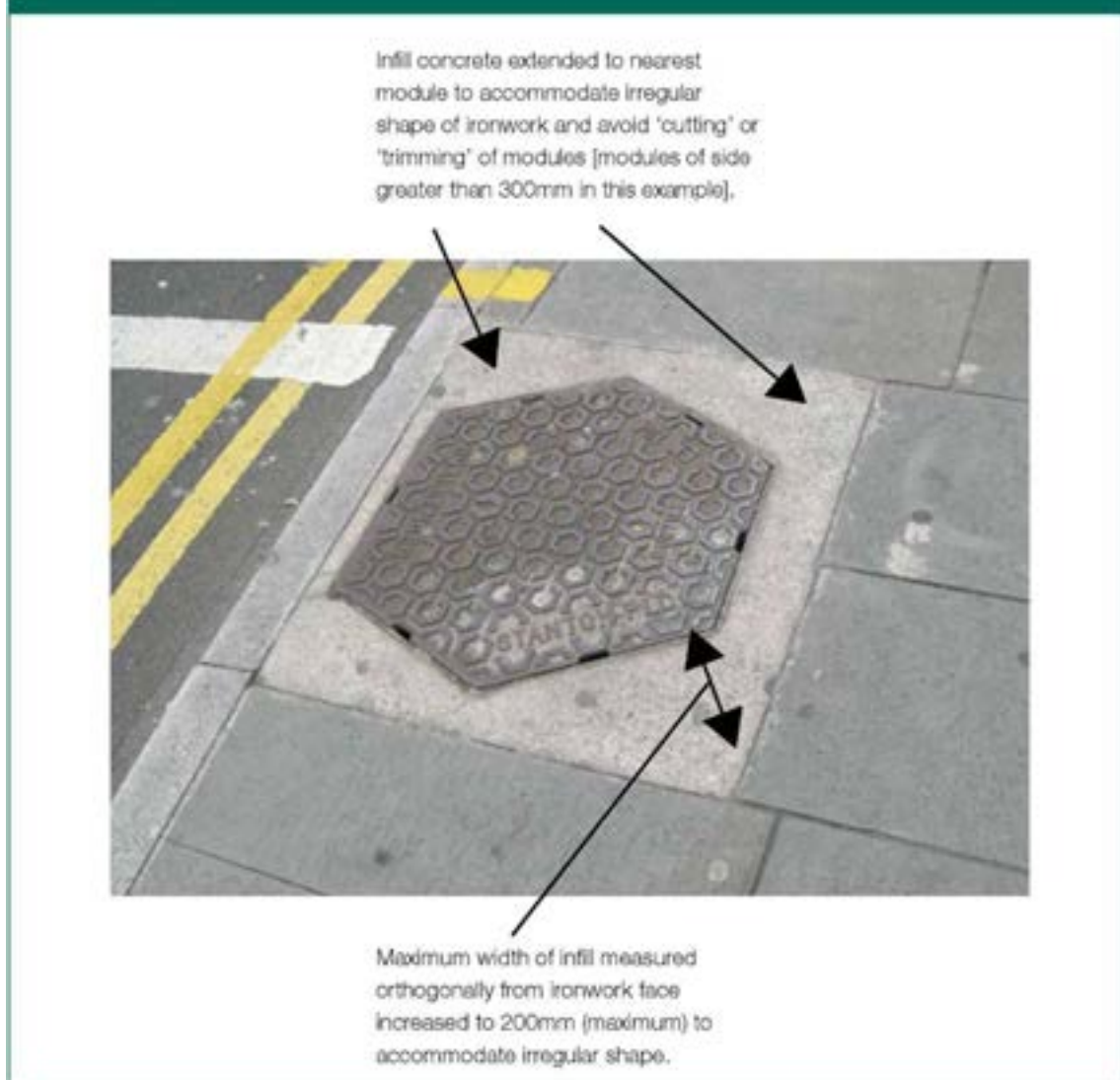
Figure NGA12.1 Extension of Infill Concrete – Modules greater than 300mm [Picture 1]
