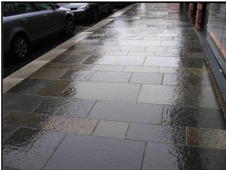
Figure 38: Good example of level footway surface
