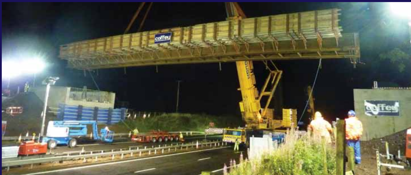
Above Replacement of the Chartershall Bridge across the M9 (© Crown copyright)
