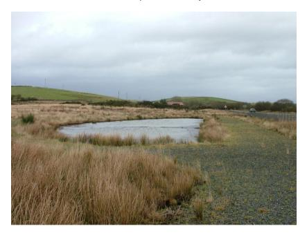
Where the Tor Bar Burn is culverted under the A75 the site visit identified an issue with drainage on site. The following plate shows that flooding is occurring adjacent to the Tol Bar Burn on the island between the two carriageways.
