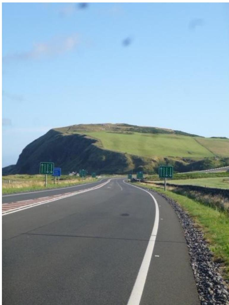
*Plate 4: view north along the scheme to its integration with the previously constructed climbing lane. View shows widened verges and the stone walls along its length*
