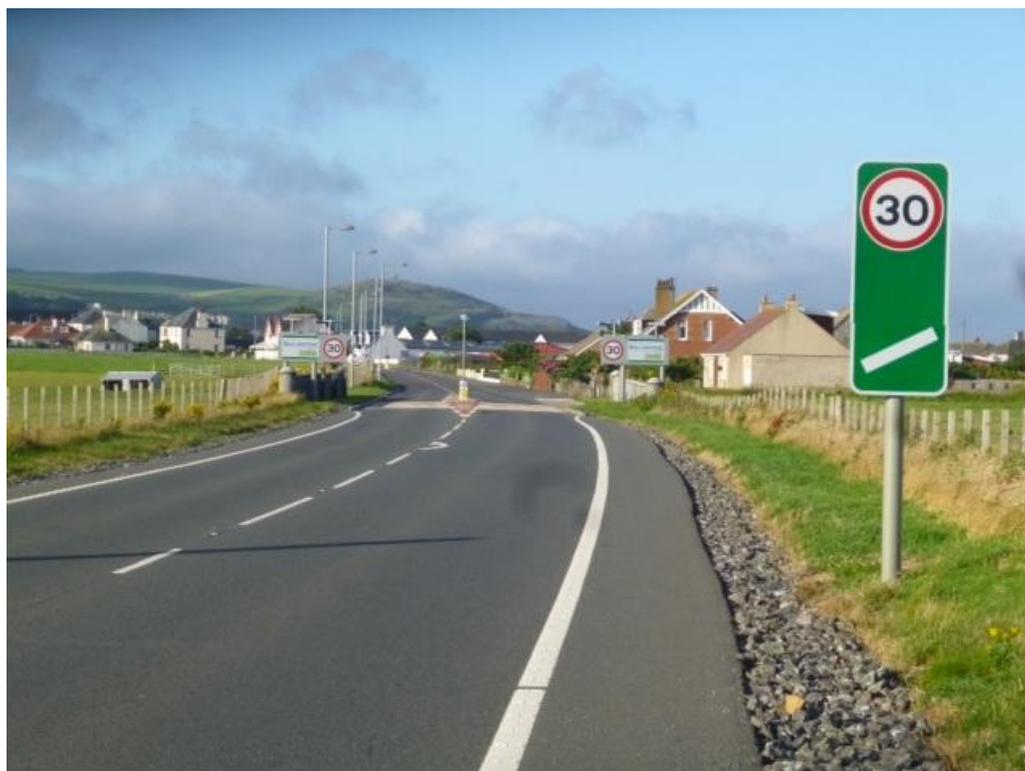
*Plate 9: Entrance to the village of Ballantrae with new speed limit signs and central island on the A77*
