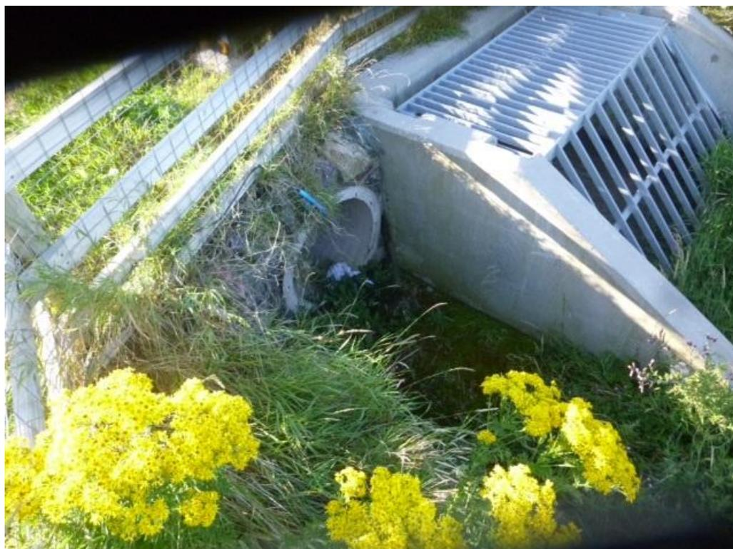
*Plate 3: Culverted watercourse with associated dry otter tunnel*
