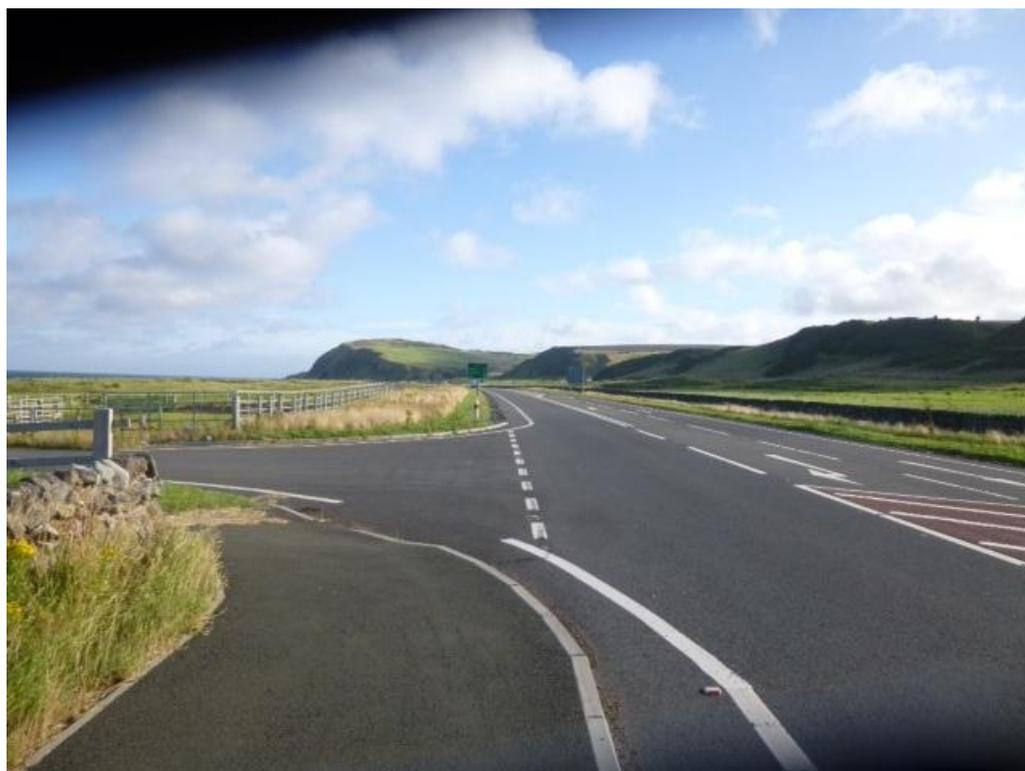
*Plate 7: New footpath on the western side of the scheme*
