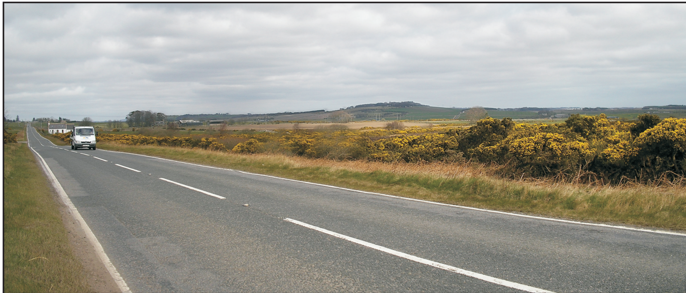
Viewpoint 3 - B979 looking North : Existing View
