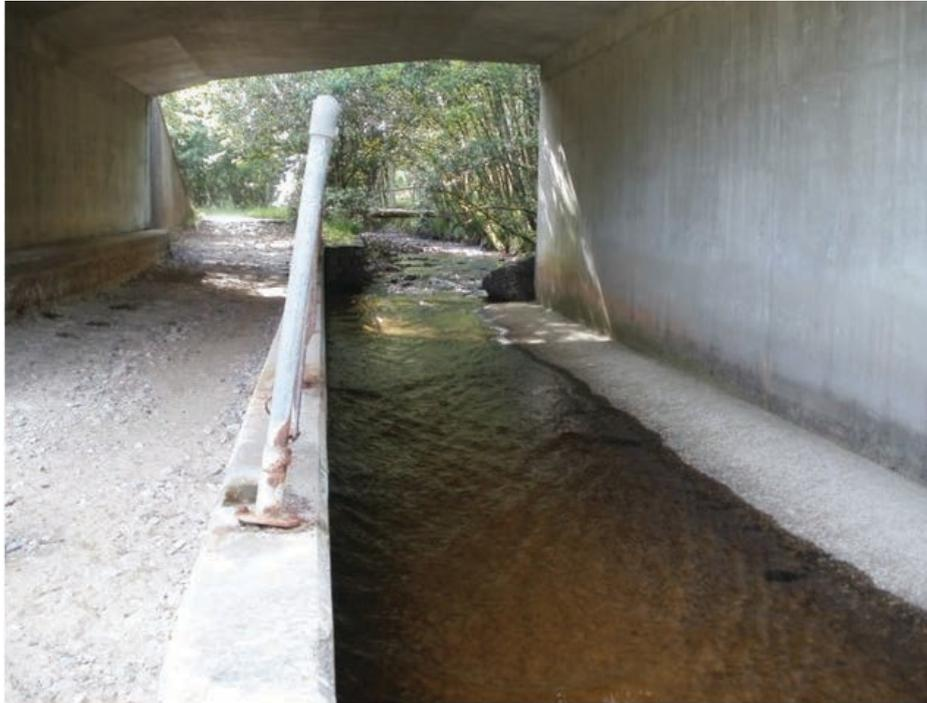
Photographs 34 & 35. Allt an Fhearna and underpass. Note trash line on fencing indicating height of spate flows. Bridge works should allow for retention of dry ledge or retro-fit ledge on north bridge abutment at a height to accommodate mean high-water levels to allow passage to mammals.
