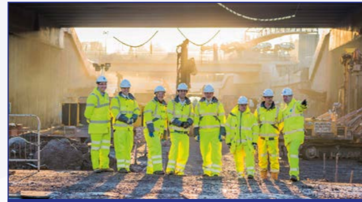
ICE UK President Prof. Broyd meets the construction team and Transport Scotland representatives at Raith underpass
