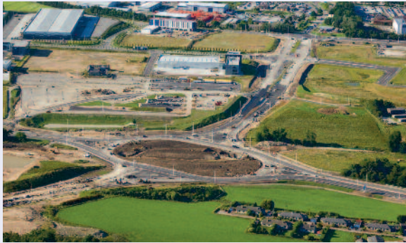
Craibstone Roundabout under construction on the A96
