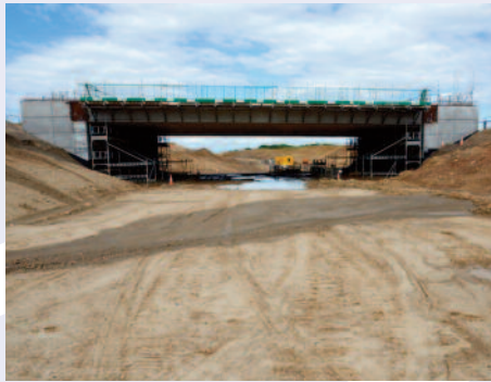
Tippetry Junction underbridge
