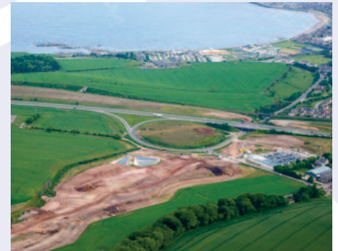
Stonehaven Junction progress
