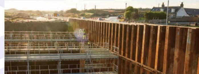
The new Balmedie Junction, which is currently under construction, will provide a grade-separated junction with connections to Balmedie and the A90 in both directions. The new junction includes roundabouts east and west of the A90, which are connected by a road passing beneath the A90 through an underpass.
