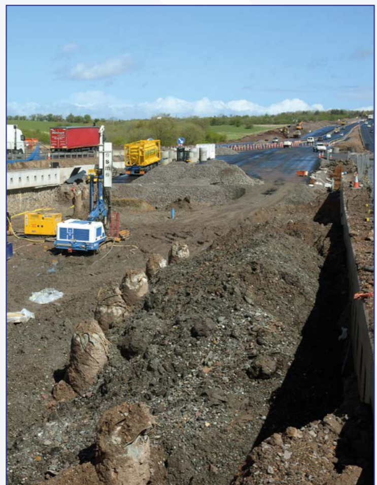
The underpass at Raith Junction taking shape
