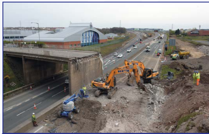
Southern half of the bridge being demolished
