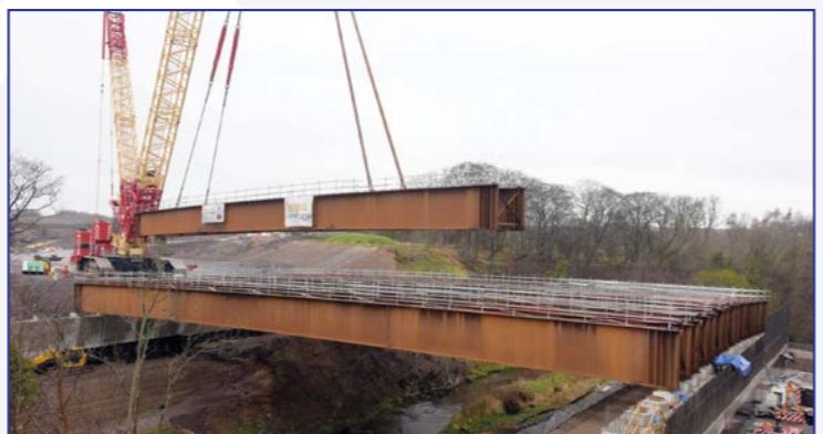
Final beam being installed
