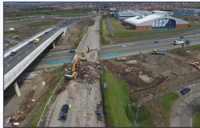
New bridge visible as old bridge is taken down
