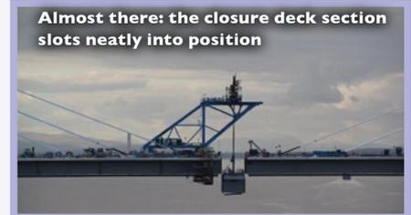
two leading edges to exactly the correct geometry. When everything is ready, we slowly release the compression on the jacks at the South Tower so that the over 600m long South Tower deck span can move back the 300mm, thus closing the gap and allowing the other side of the closure section to be welded and concreted into position. When this is complete, full closure has been achieved.
