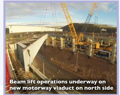
**Beam lift operations underway on new motorway viaduct on north side**
