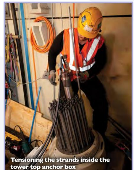
Tensioning the strands inside the tower top anchor box
