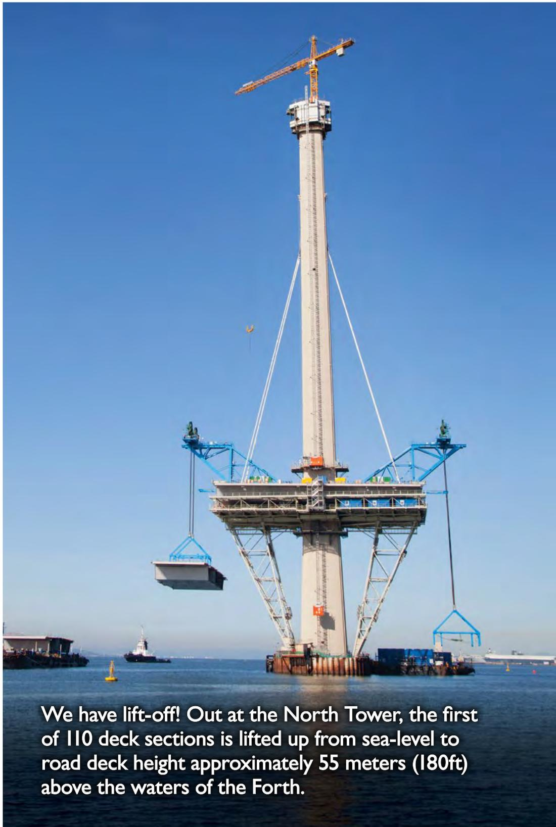
We have lift-off! Out at the North Tower, the first of 110 deck sections is lifted up from sea-level to road deck height approximately 55 meters (180ft) above the waters of the Forth.
