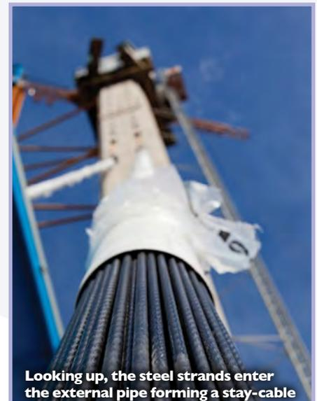
Looking up, the steel strands enter the external pipe forming a stay-cable
