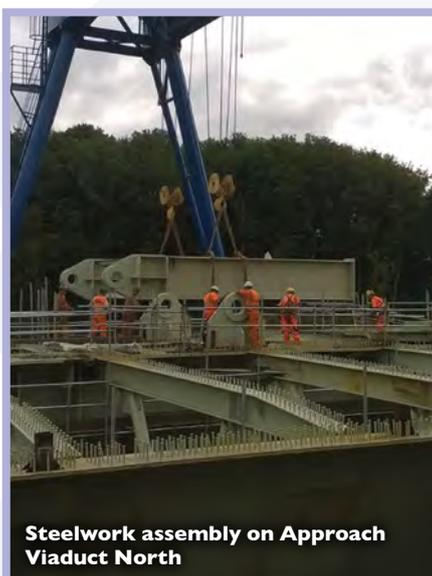
**Steelwork assembly on Approach Viaduct North**
