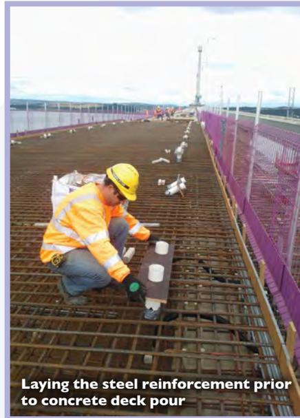
**Laying the steel reinforcement prior to concrete deck pour**
