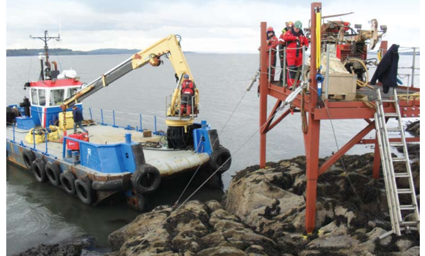
Temporary platform on Beamer Rock.
