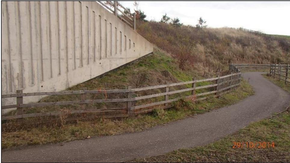
**Figure A.3: Missing section of the mammal fence by the underpass at Bellyford Burn**
