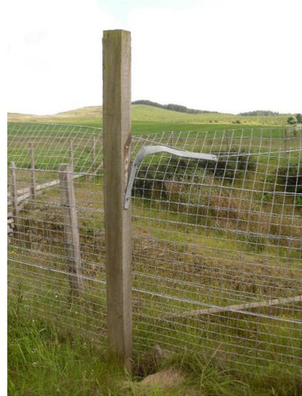
*Figure 8: Damaged fence post in mammal fence*
