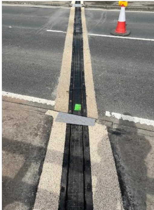
A83 Fyne Bridge Joint Replacement
