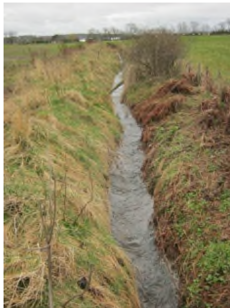
Plate 9: Straight planform and trapezoidal cross-section of SWF 08
