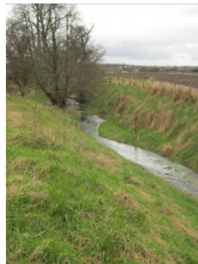
Plate 4: Embanked channel downstream of railway
