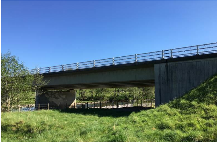
Photograph 9.19: Pitaldonich Underbridge location of existing crossing point CP12, Path 124
