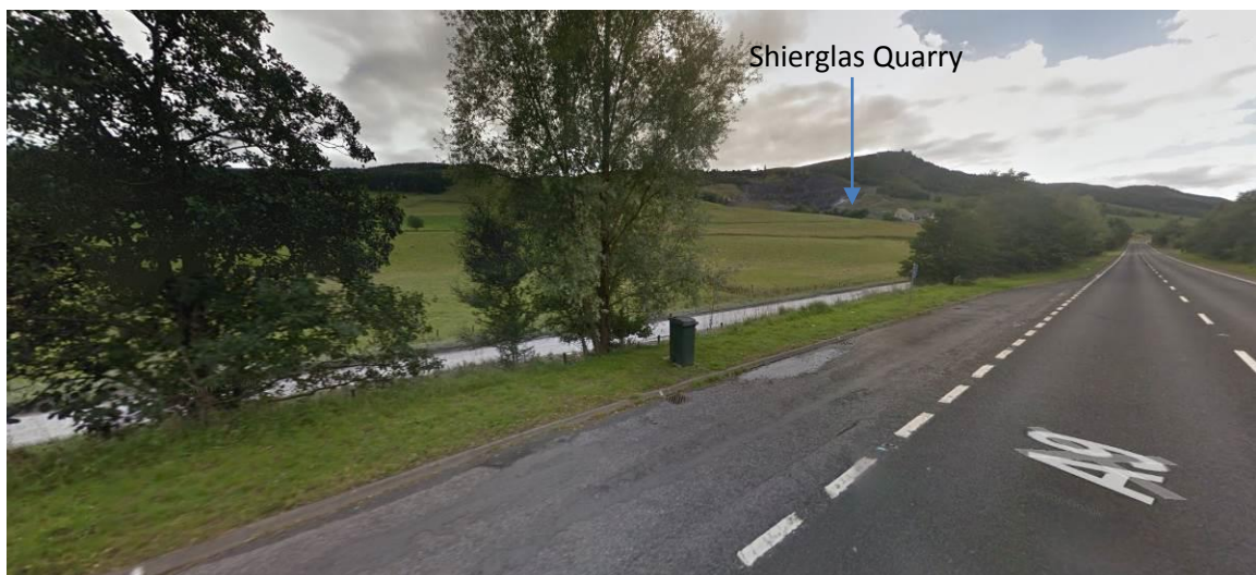
Photograph 9.30: Lay-by Ref no 3, northbound view
