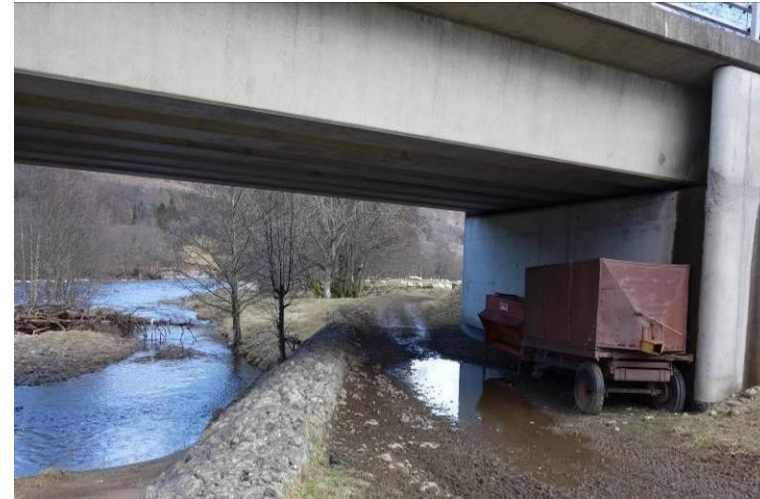
Photograph 9.18: Pitaldonich Underbridge location of existing crossing point CP11 (Paths 120 and 121 shown)
