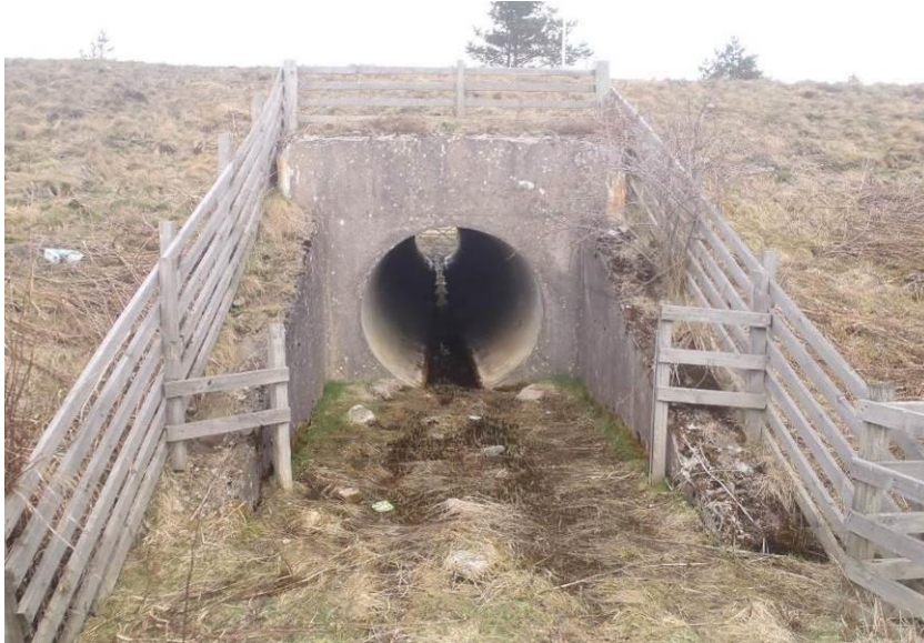
Photograph 9.25: Existing non-vehicular underpass to the west of Tigh-na-Collie using Path 137 (CP18)
