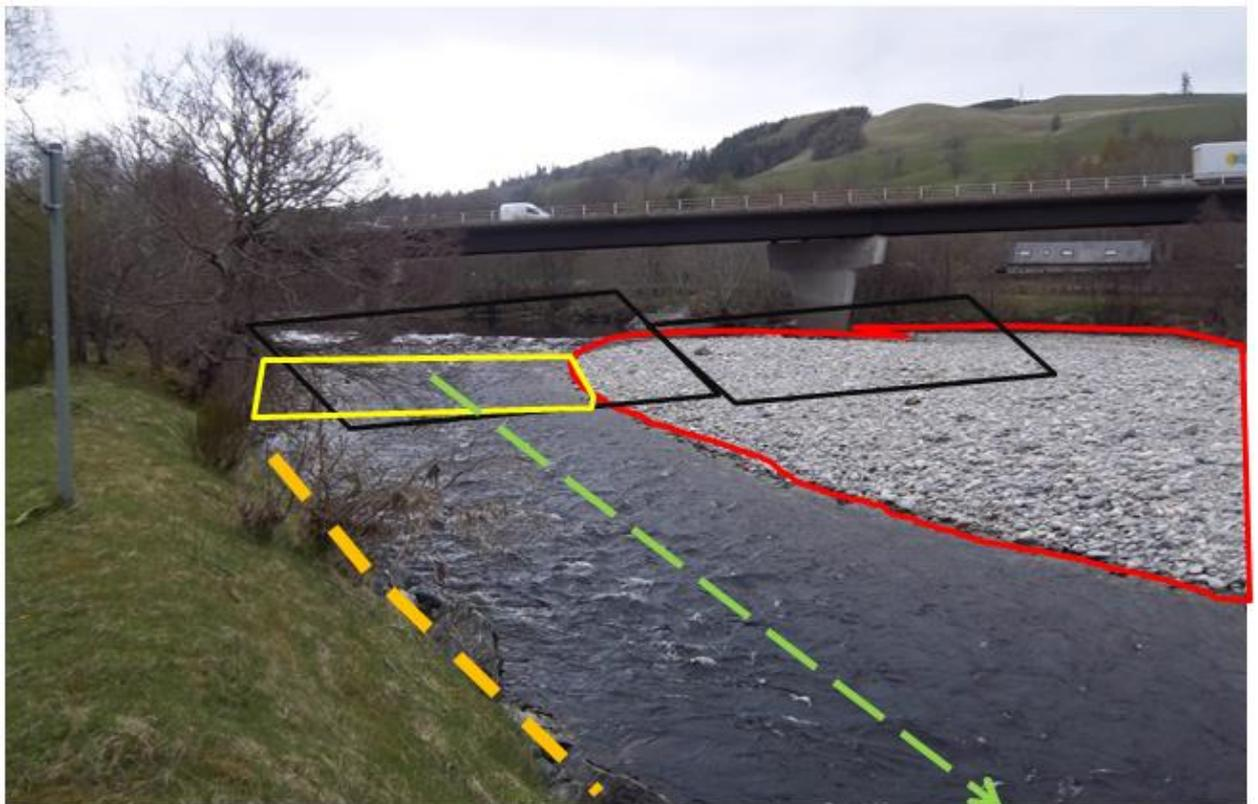
8.1.15 Figure A11.8.9 (in Appendix A11.8: Watercourse Crossings Report) and Diagram 3 below provide a more detailed schematic plan of the potential channel change around the bridge piers and the consequent downstream adjustment. This may include the potential for:
