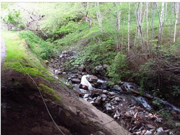
**Photograph 10: Collapsed gabion baskets in channel (looking downstream)**
