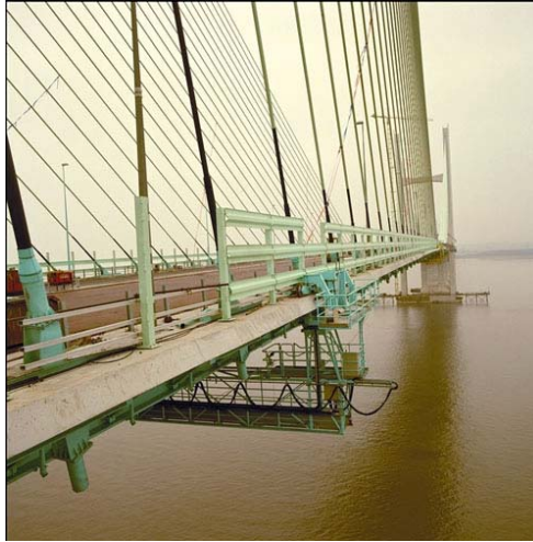
Figure 3: Second Severn Crossing Windshielding under construction
