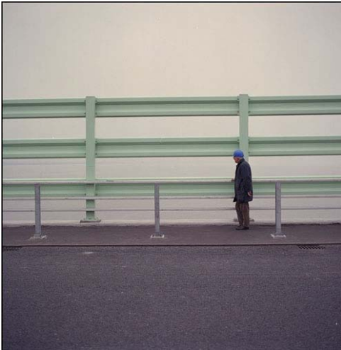
Figure 2: Second Severn Crossing Windshielding – Approach Spans
