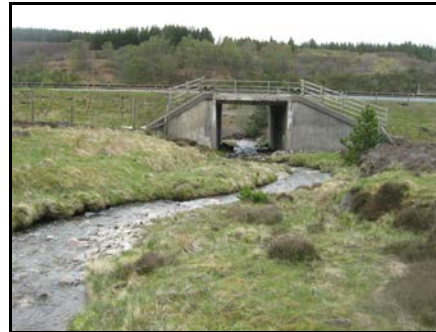
b) Upstream view looking at A9 from the east
