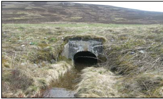
a) Downstream of the A9 looking east toward road
