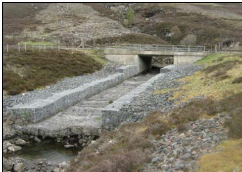
a) Downstream looking east toward A9
