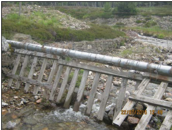
a) Upstream view east of A9, showing areas of sediment deposition adjacent to channel realignment
