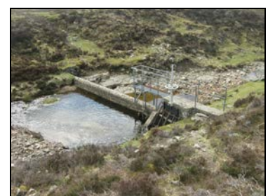
c) Dam upstream of A9 crossing (ABS8.8)
