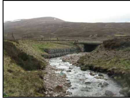
b) Upstream view looking at A9 from the east
