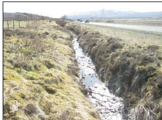
b) Upstream of the A9 looking south
