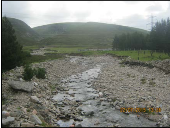
a) Upstream view east of A9, showing areas of sediment deposition
