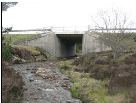
a) Downstream looking at A9 from the west
