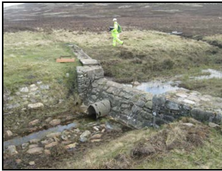
a) Dam east (upstream) of the A9 (ABS8.7)
