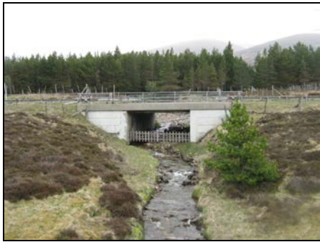
a) Downstream looking at A9 from the west
